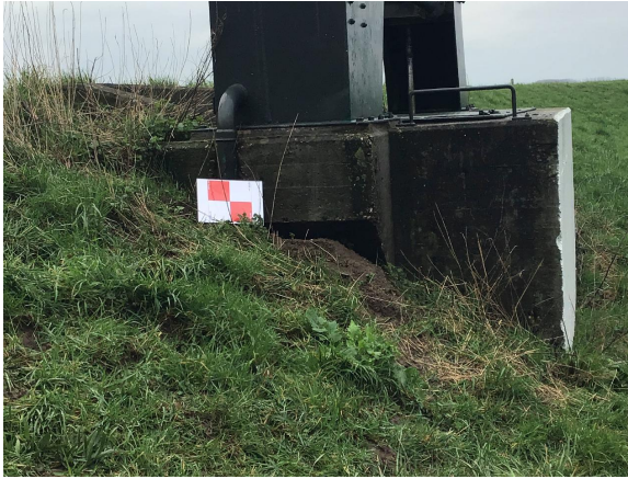
Figure 6.9.: Example of the presence of multiple damage parameters at a single damage point (4_3). At least bare spots, weeds and rough vegetation could be applicable here, while the cause of the bare spot (just right of the reference marker) could be burrowing.
