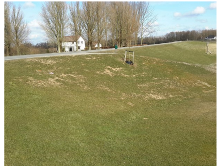
(d) Bad: > 6 spots with diameter > 0.2 m, or 1 spot with diameter > 0.3 m where vegetation is gone.
