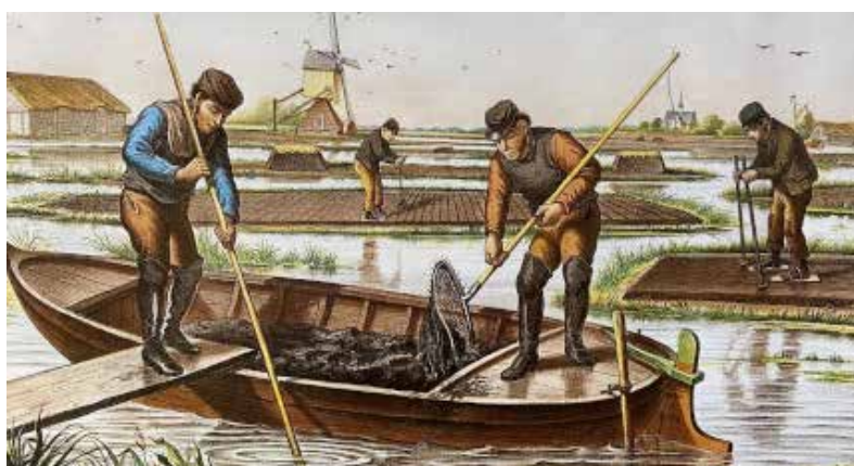
Figure 4 - Dredging with a baggerbeugel in the 16th century
