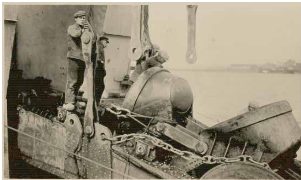
Figure 5 - Repair of bucket dredger HAM 107 Pernis, showing the grandeur of the new dredging machinery
