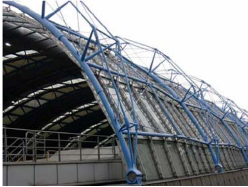
Figure 2 Telescopic steel tubes in Waterloo International Railway Station
