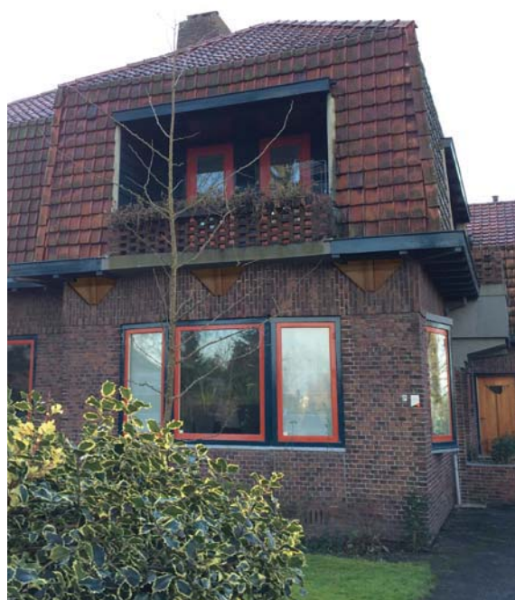
Figure 188: After retrofit, source: own elaboration
