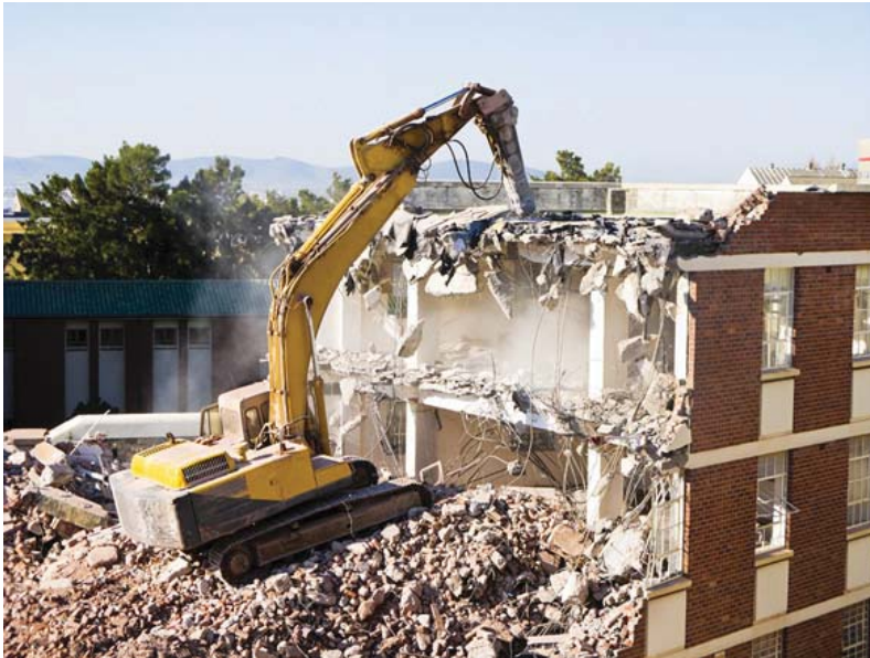
Figure 39: Demolition source: www.powell-constructors.com
