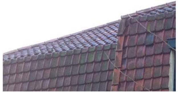
Figure 91: Ceramic roof tiles, source: own elaboration
