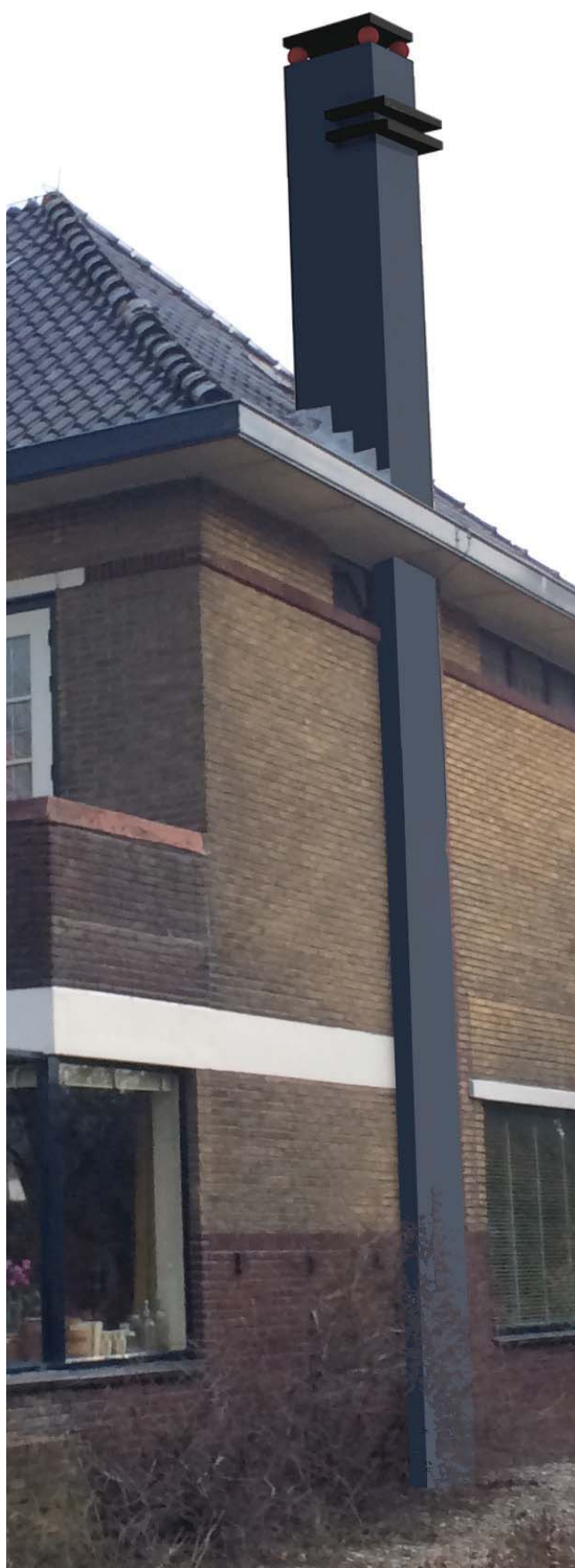
Figure 152: After retrofit, source: own elaboration
