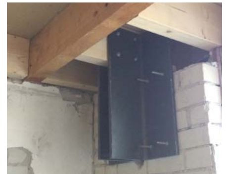
Bolted beam shoe
