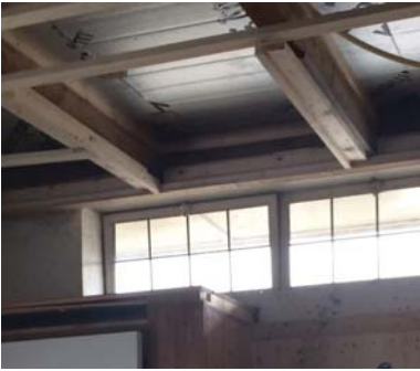
Figure 111: Wooden beams, Source: own elaboration
