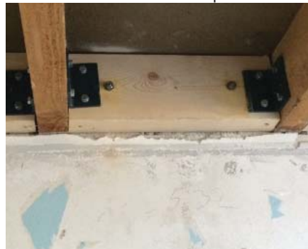
Bolted and glued steel profile
