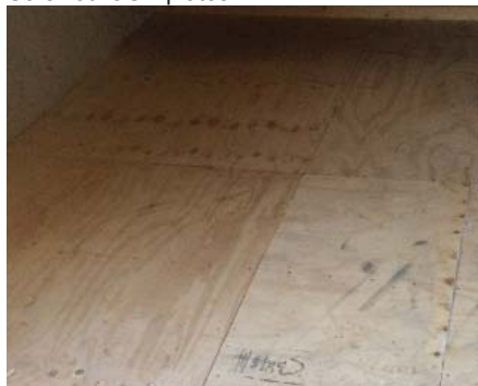
Figure 120: Test houses diaphragm stiffening, source: own elaboration
