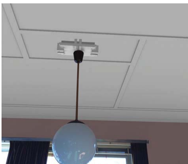
Figure 212: After retrofit, source: own elaboration
