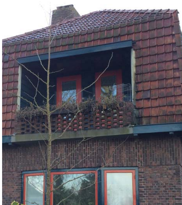
Figure 171: Before retrofit, source: own elaboration
