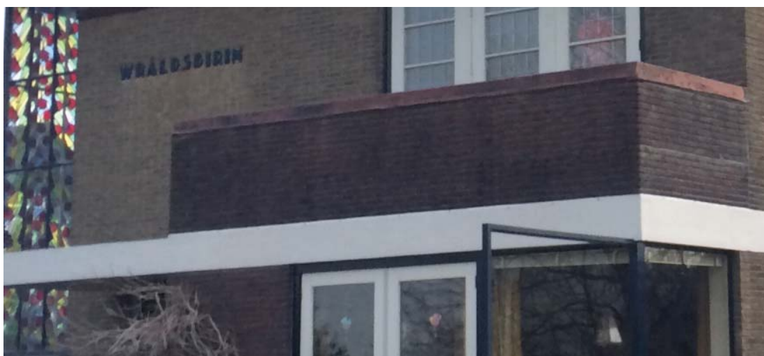
Figure 158: Before retrofit, source: own elaboration
