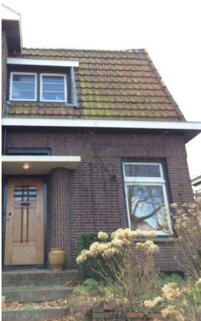
Figure 194: Before retrofit, source: own elaboration
