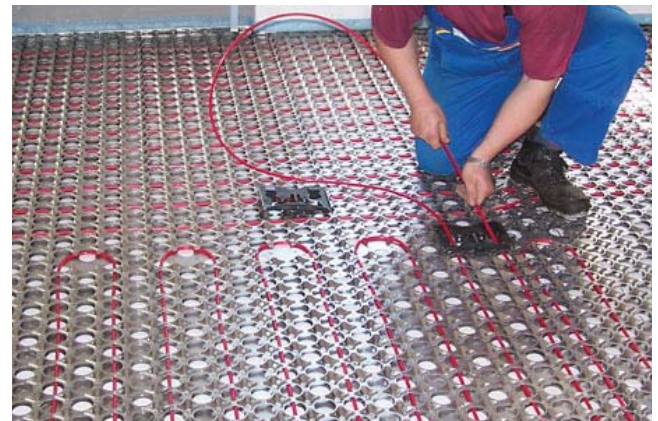
2. Installation of the floor heating
