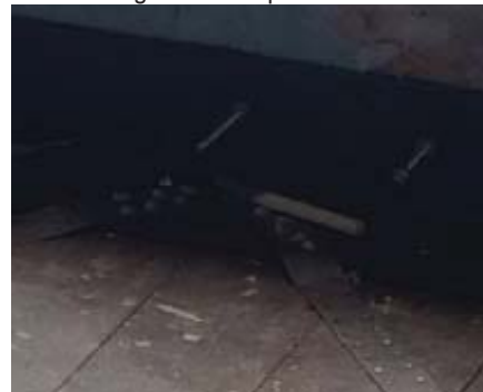
Figure 121: Test houses floor-wall connections, source: own elaboration
