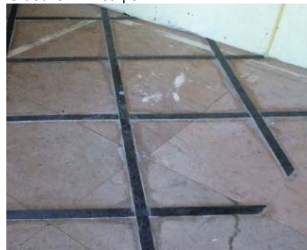
Figure 120: Test houses diaphragm stiffening, source: own elaboration
