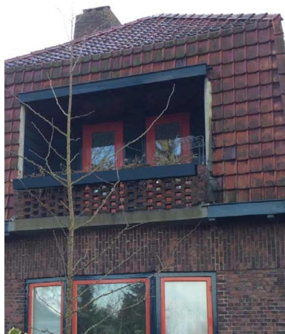
Figure 172: After retrofit, source: own elaboration
