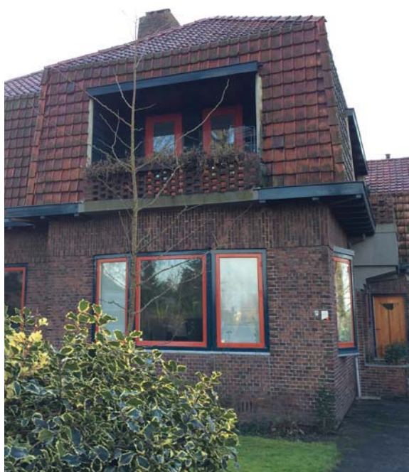
Figure 187: Before retrofit, source: own elaboration
