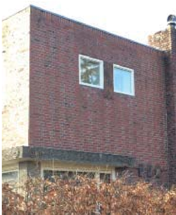
Figure 182: Before retrofit, source: own elaboration
