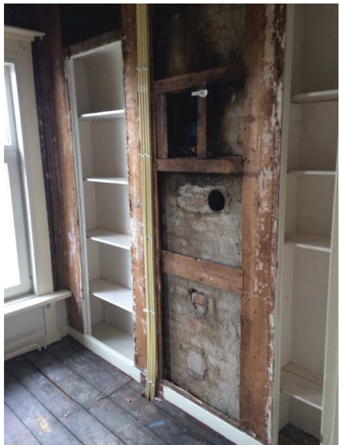
Figure 123: Removed chimney in test house, source: own elaboration
