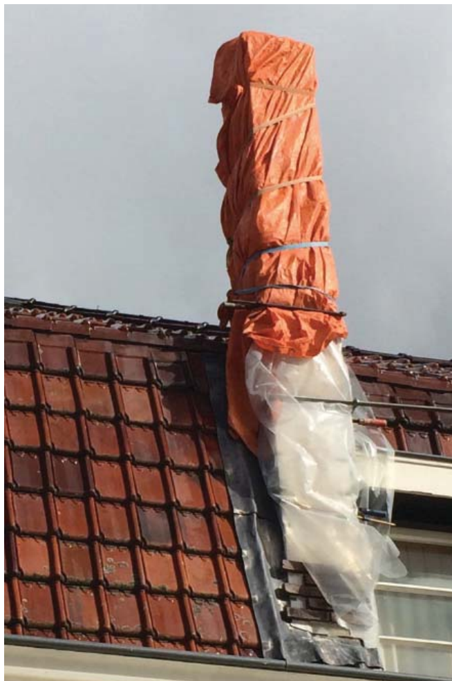
Figure 106: Replacement of a chimney, Wijmerspad 1, Source: own elaboration
