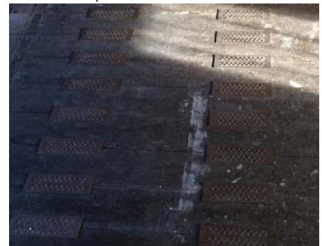
Nailed steel strips
