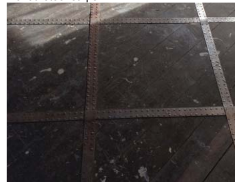
Nailed steel strips
