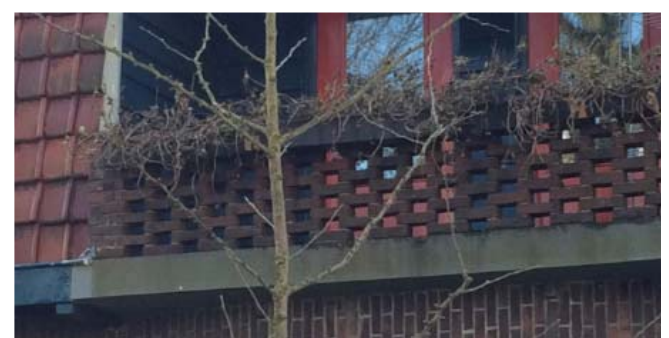
Figure 89: Masonry parapets, source: own elaboration
