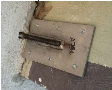
Bolted and glued steel profile
