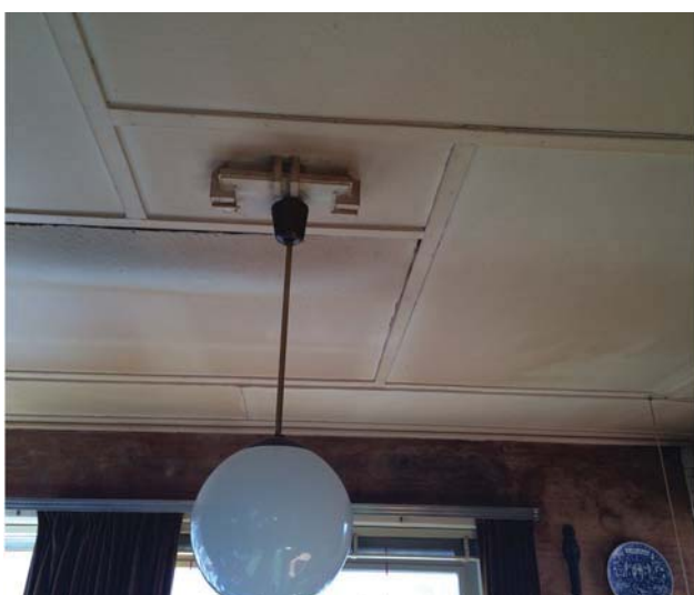
Figure 211: Before retrofit, source: own elaboration
