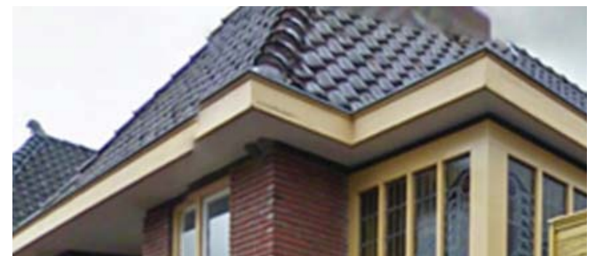
Figure 87: Box gutters, source: own elaboration
