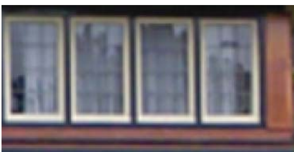
Figure 73: Strip windows, source: own elaboration
