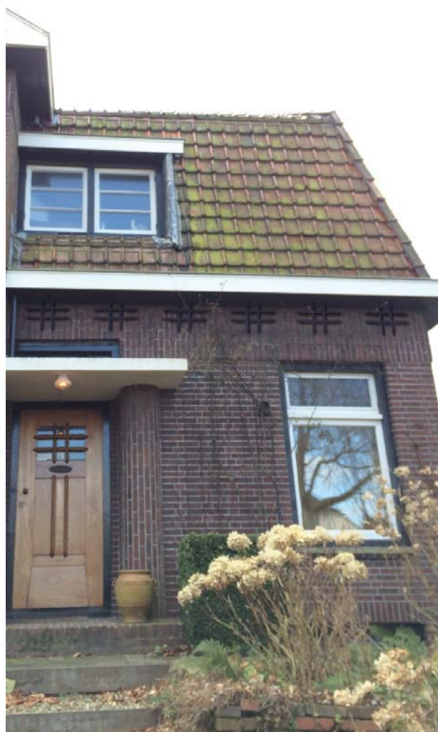
Figure 195: After retrofit, source: own elaboration
