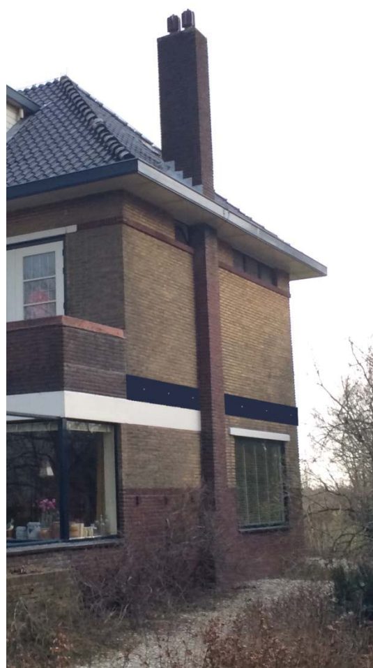
Figure 201: After retrofit, source: own elaboration
