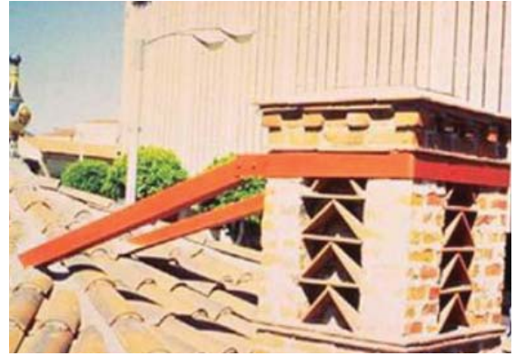
Figure 31: Chimney restraint, source: Arup, 2013
