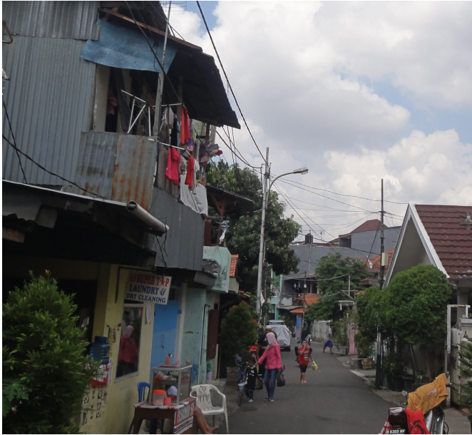
Brick ground floor, sheet metal first floor
