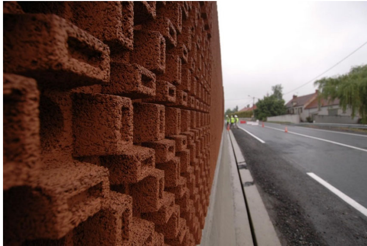
Figure 32: Fractals inspired acoustic sound absorption design (source: Wan et al., 2020)
