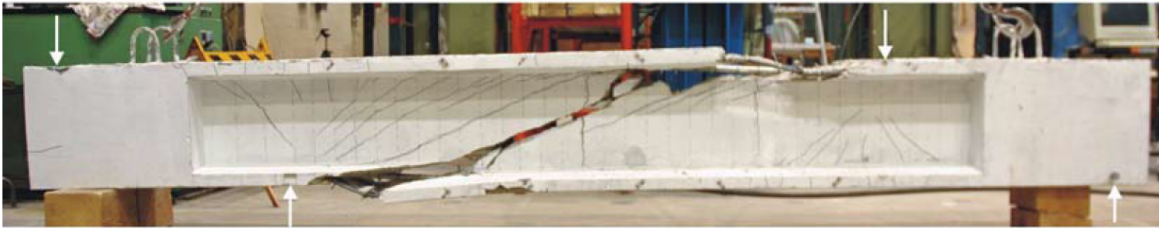
Figure 3-8: Failure of beam LB10 [13]; A_s = 934\text{mm}^2 , N = -822\text{kN} , V_u = 215\text{kN} , s = 87.5\text{mm}
