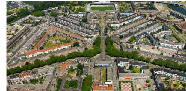
Figure 5.1.2.2: Aerial view from South of Spangen neighbourhood (Source: https://www.aerophotostock.com/media/b0ac62f2-cc04-4dec-99d5-97399b366851-spangen-rotterdam-nederland-30-juni-2015-spangen-is-eenwijk ).
