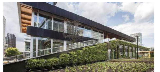
Figure 4.4.4.1: Lateral side of the pavilion, where local food production can be freshly harvested (Source: https://www.bambouwentechniek.nl/projecten/circl-circular-paviljoen-abn-amro-amsterdam?position=2&list=Bi95qLZ6fxmNr7jxHefdGXDB_vz54rXSUULlgEXDgOU ).
