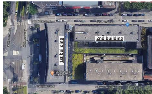
Figure 6.3.4.1: Current situation of the two rooftop possible locations for the greenhouse (Source: Google Maps). ☉ N
