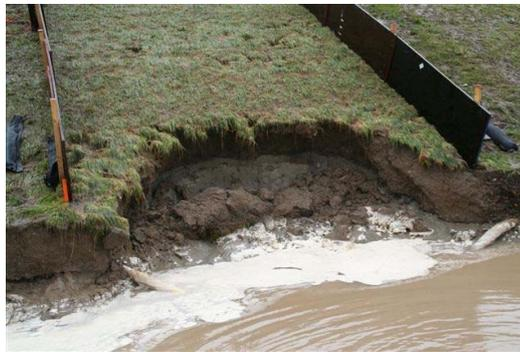
**Figure 2 Extensive damage at maintenance road at the transition slope to horizontal at the toe with progressive head-cut erosion**
