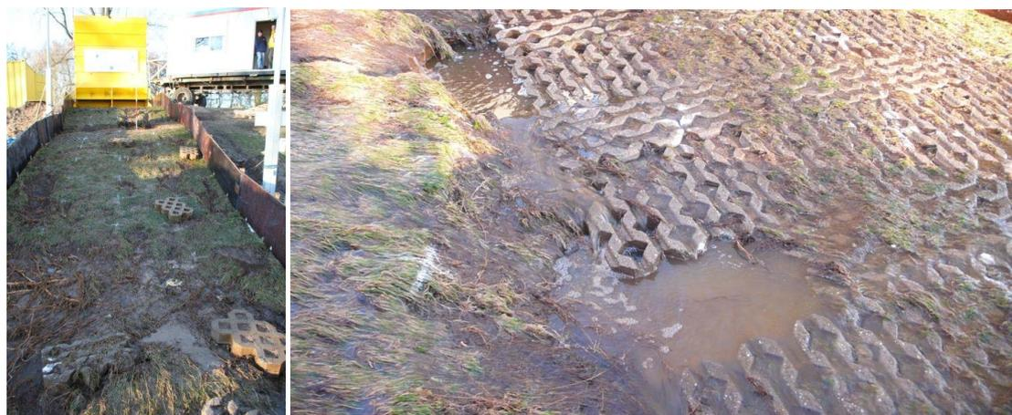
**Figure 4 Damaged open concrete block pavement on a berm (left: removed blocks on the downstream slope; right: initial scour hole development at the upstream side of the pavement)**
