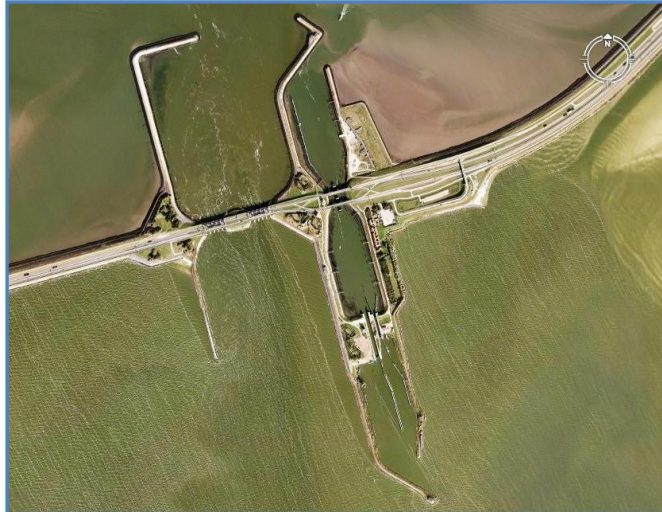
Figure 2-5: Lock-slucice complex Kornwerderzand, Friesland (Google Earth, 2008)
