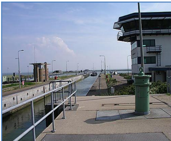
Figure 4-1: Old (left) and new (right) control towers at Kornwerderzand.
