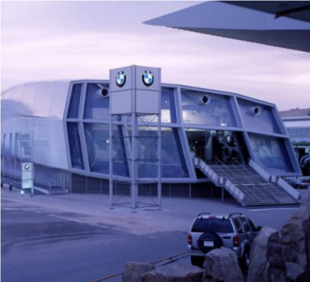
Fig. 74 BMW Dynaform pavilion, ibz+L, Bollinger + Grohmann, Frankfurt, Germany, 2001
