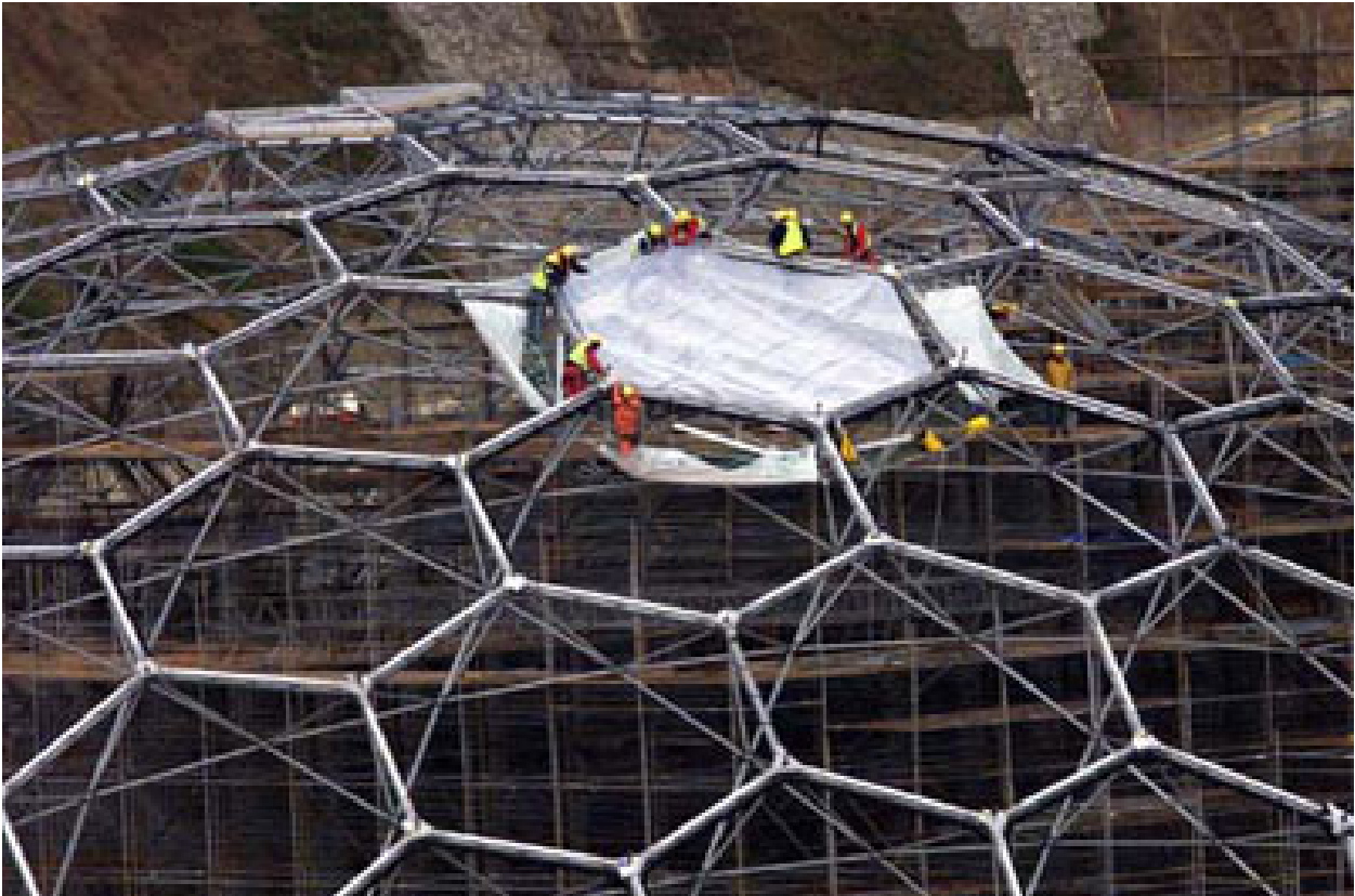
Fig. 60 Eden project under construction
