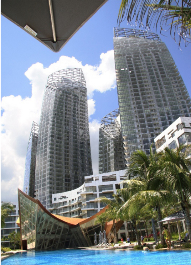
Fig. 96 Reflections at Keppel bay, Studio Daniel Libeskind & DCA architects, Singapore, Republic of Singapore, 2011
