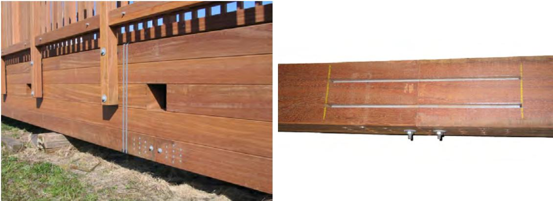
**Figure 1-1: Azobé bridge in the Netherlands with detail of joint (fotos: J.W.G. van de Kuilen)**
