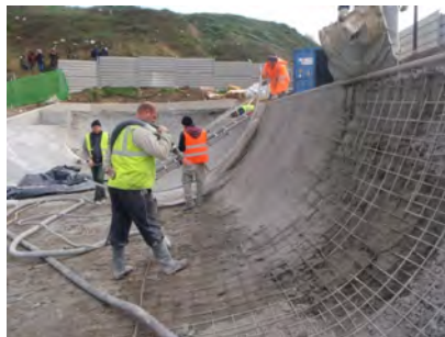
Figure 2.8: Spraying concrete on curved surface (confuzine.com)
