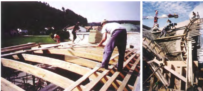
Figure 2.1: Timber formwork construction and casting of Isler shells (taken from Bösigler, 2011)
