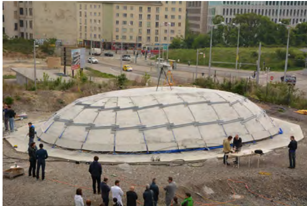
Figure 2.5: Thin concrete elements lifted by inflation of a pneumatic formwork (TU Wien, 2014)
