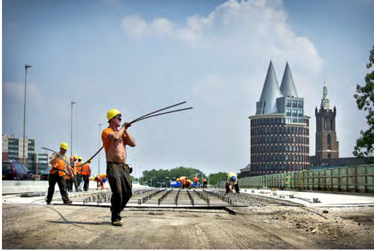
Figure 8.9: The natural deflection of steel bars - clearly visible here - is a function of diameter, self weight and support positions (Maasbrug Roermond, image Peter Wijnands Photography)
