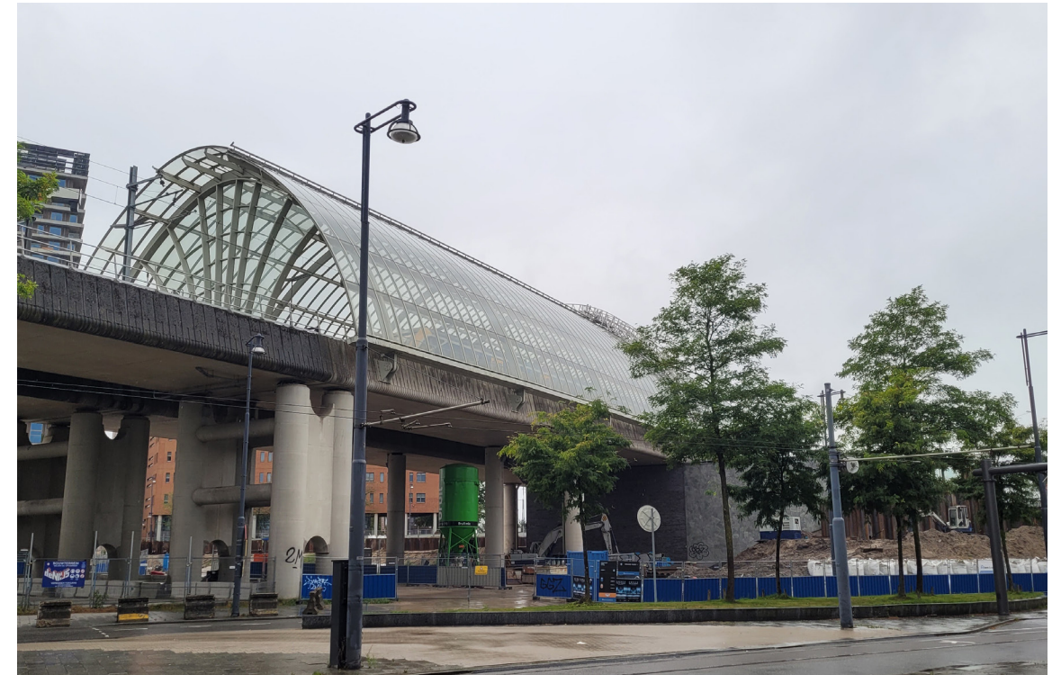
Figure 42: Picture taken in Sloterdijk Station Area
