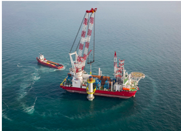
Figure 1.4: Seajacks Scylla installing a monopile [Seajacks, 2018]
