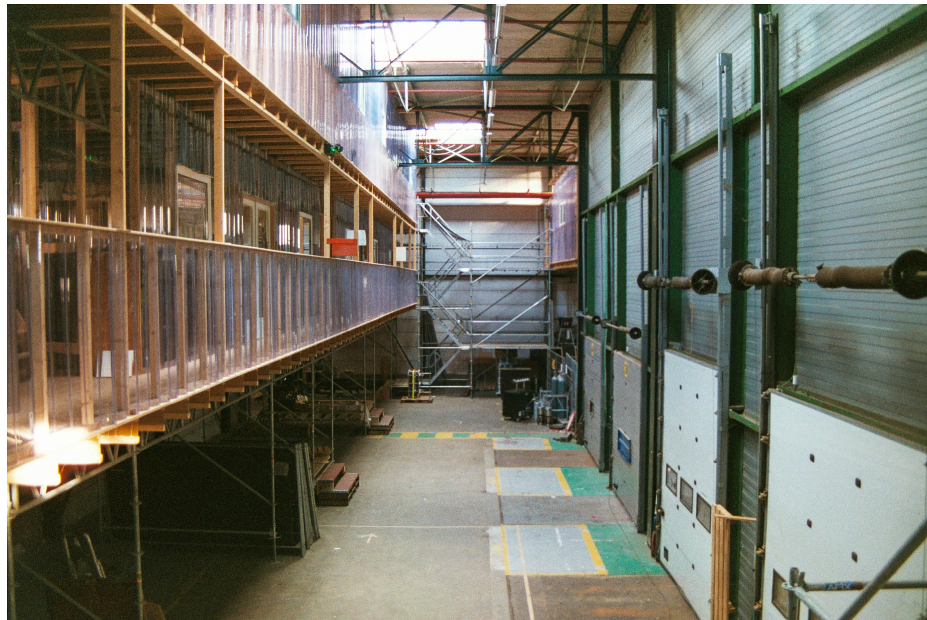
Ateliers and indoor street in Blikfabriek. Photo by author
