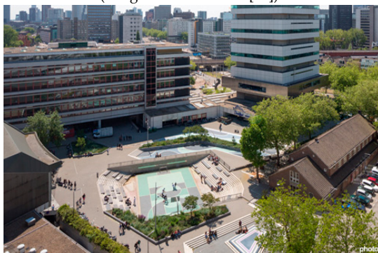
(e) Benthemplein Water Square (image retrieved from [35])
