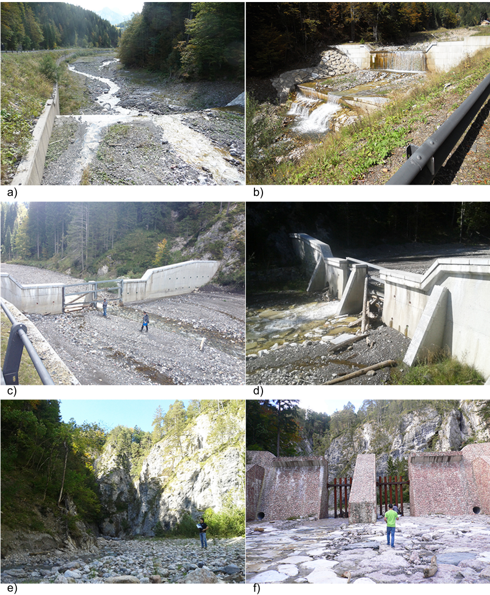
Figure 4.3: Photos of the structures inspected: (a) downstream view of check dam 1; (b) check dam 1 and sill structures located in series; (c) downstream view of check dam 2; (d) level of obstruction in check dam 2; (e) upstream deposit in check dam 3; and (f) level of obstruction in check dam 3.
