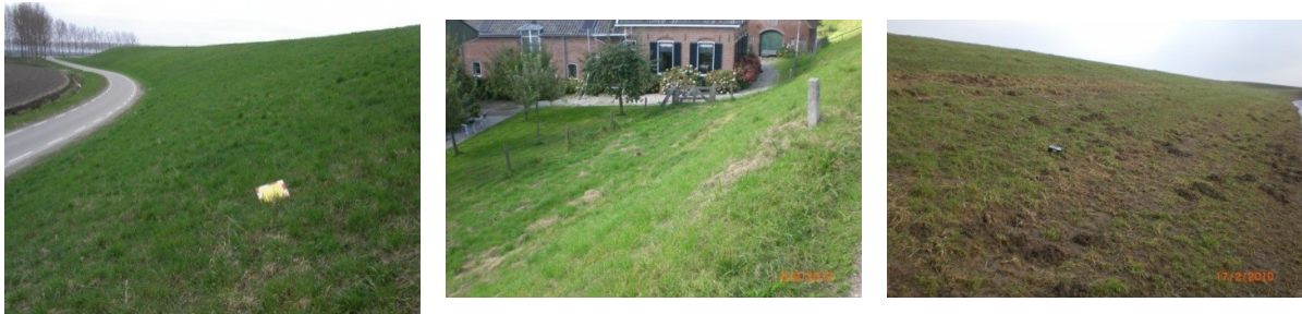
Figure 2.2: Examples of references picture for different grass condition. The grass condition of the left picture is in the closed state; the middle is an open condition, and the right is the fragmented condition. Images are taken from Het Waterschapshuis (2016)
