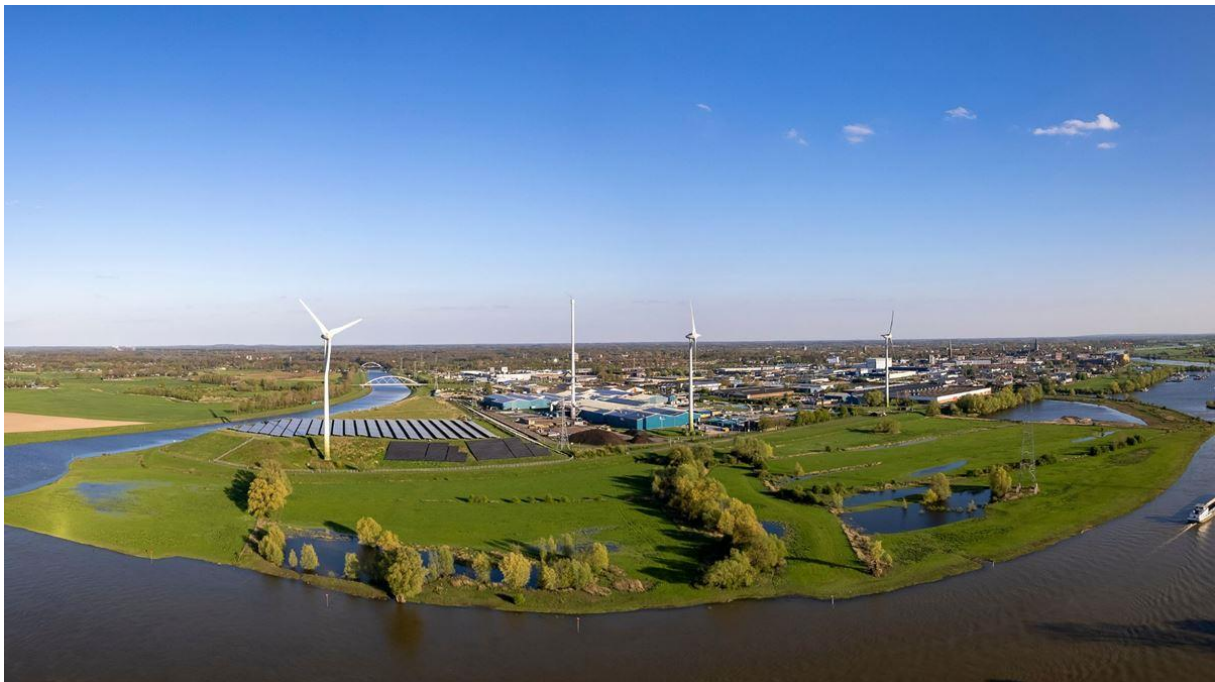
Figure 23. Smart Energy Hub at Business Park “De Mars”, Zutphen, The Netherlands (Haskoning, n.d.-b).
