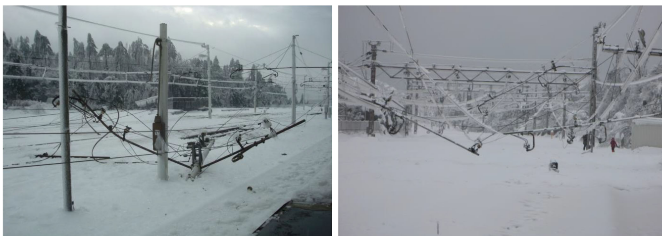
FIGURE 9 Damaged overhead lines and equipment during heavy icing in 2014, Slovenia (Gavin, 2016)
