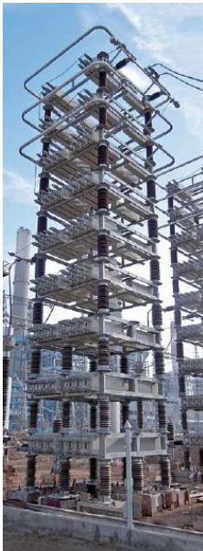
Figure 4.8: HVdc ac-side capacitor bank [100].
