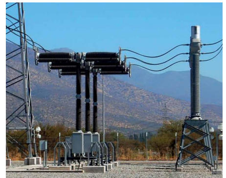
Figure 4.4: High-voltage ac circuit breaker [95].
