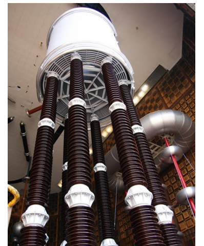
(b) VSC-HVdc phase reactor [103]
