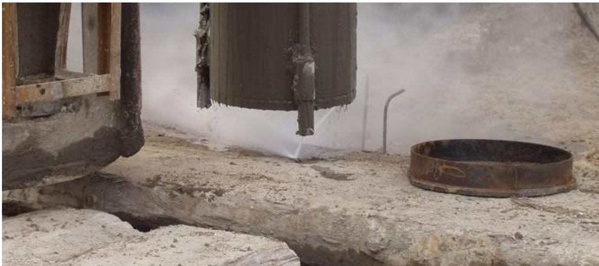
Figure 2-4: Casing of a vibro-fluidization pile with the 'drill bit' next to it (joostdevree.nl)
