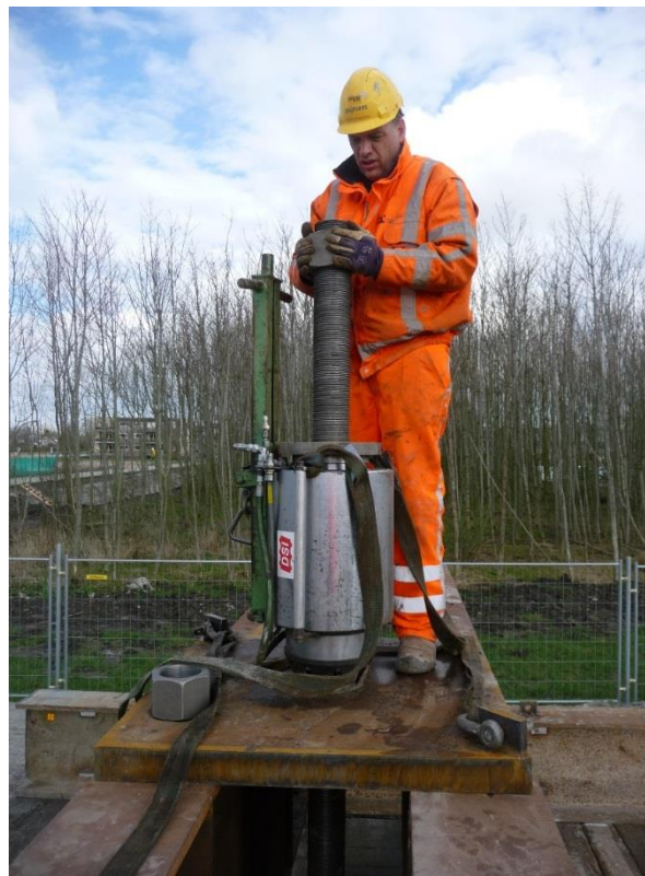
Figure 2-8: Installation of the jack (Pictures Ir. J. Kimenai)
