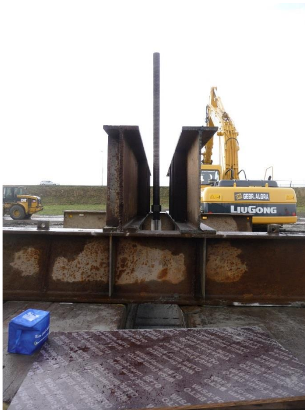
Figure 2-7: Construction to redistribute the test load towards the soil (Pictures Ir. J. Kimenai)
