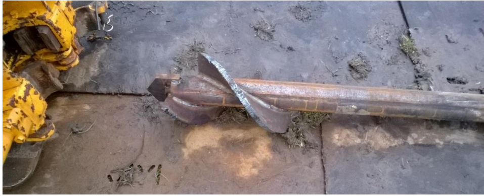
Figure 2-3: Screw blade of a Type D micropile as applied at the Drachtsterweg (Pictures Ir. J. Kimenai)
