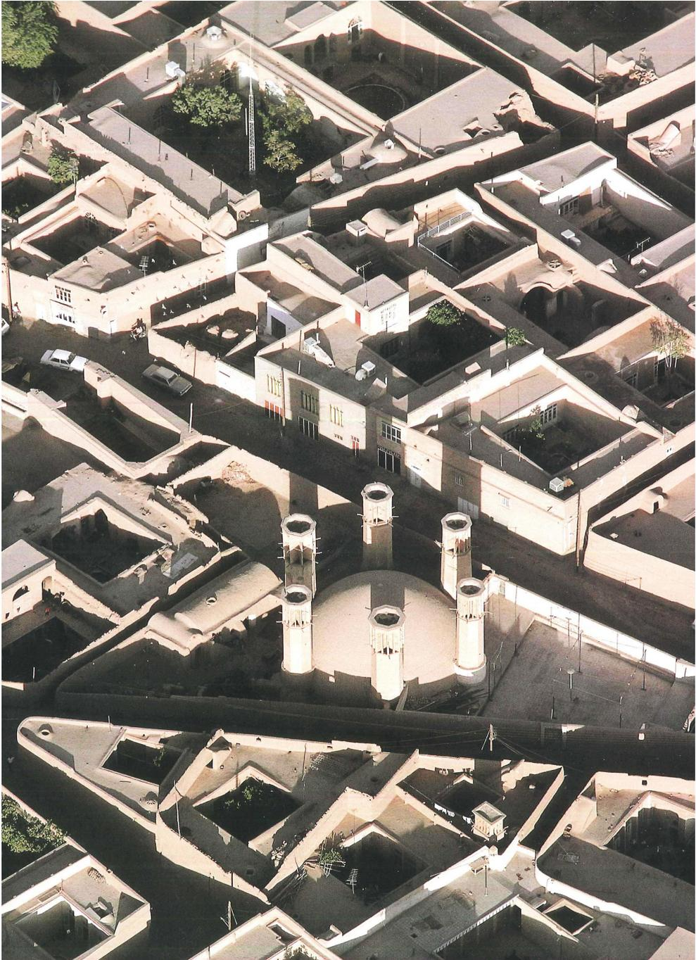
3.11: Yazd, Iran. The picture illustrates an *ab-anbar* (water storage) or domed cistern ringed by six tall wind-catchers, each of which was designed to capture the wind from all directions, for ventilation and to cool down the water. In its foundation, a perimeter wall protects the base of the dome of ab-anbar and also guides the run-off after the occasional heavy rainstorm into the cistern. Aerial photograph by Georg Gerster, 1976-78.
