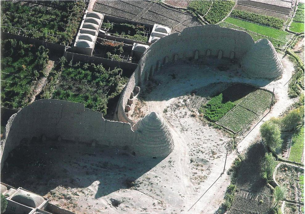
3.12: Sirjan. The picture shows an ice-making and storage structure or yakhchal. Two tall curved walls are used to provide shade for the shallow tanks, 'where, in winter, qanat water was turned into ice, chopped out and then stored in deep pits beneath the stepped, domed ice houses.'
