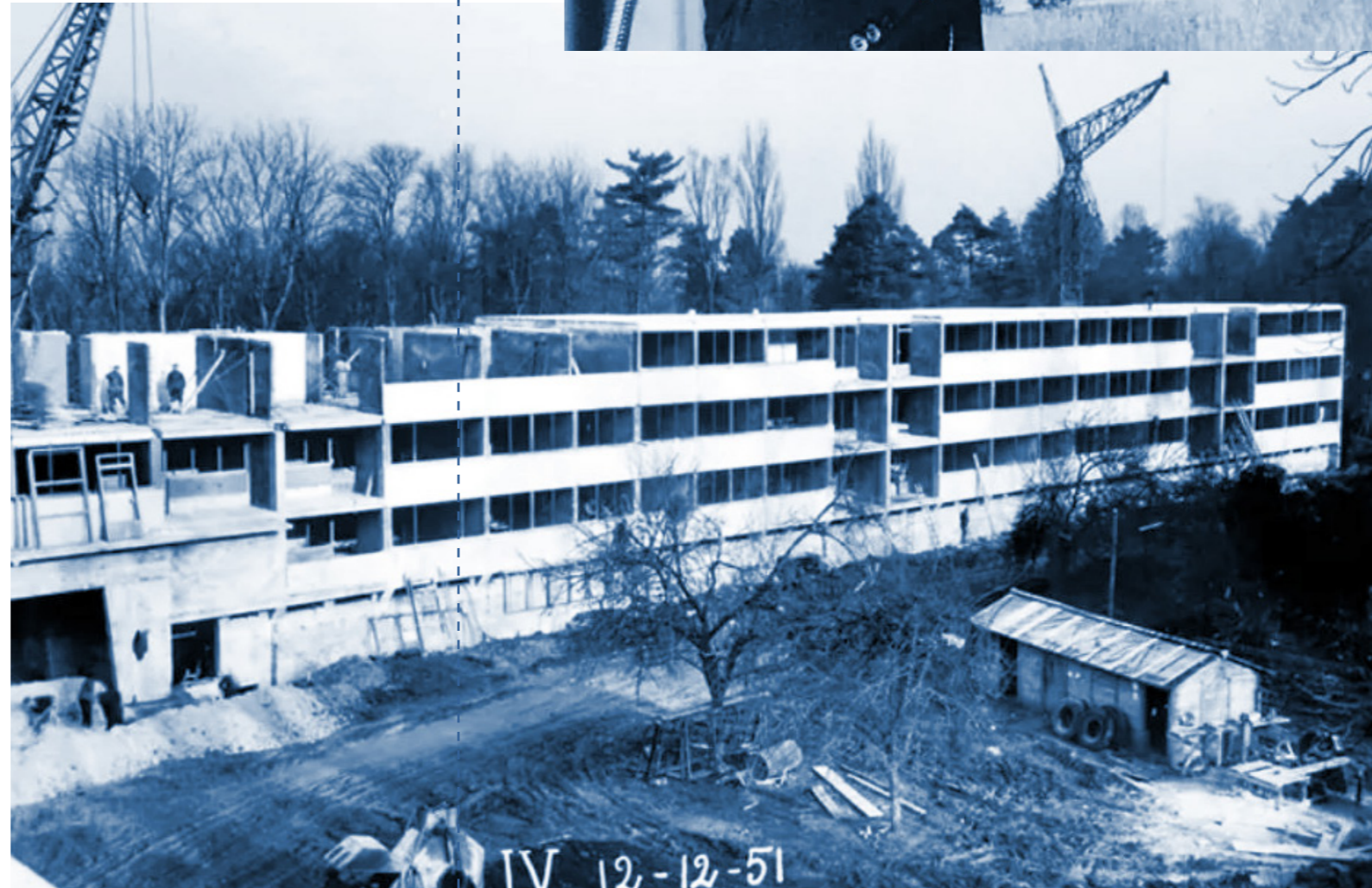
Camus' prefabricated building under construction, 1951
