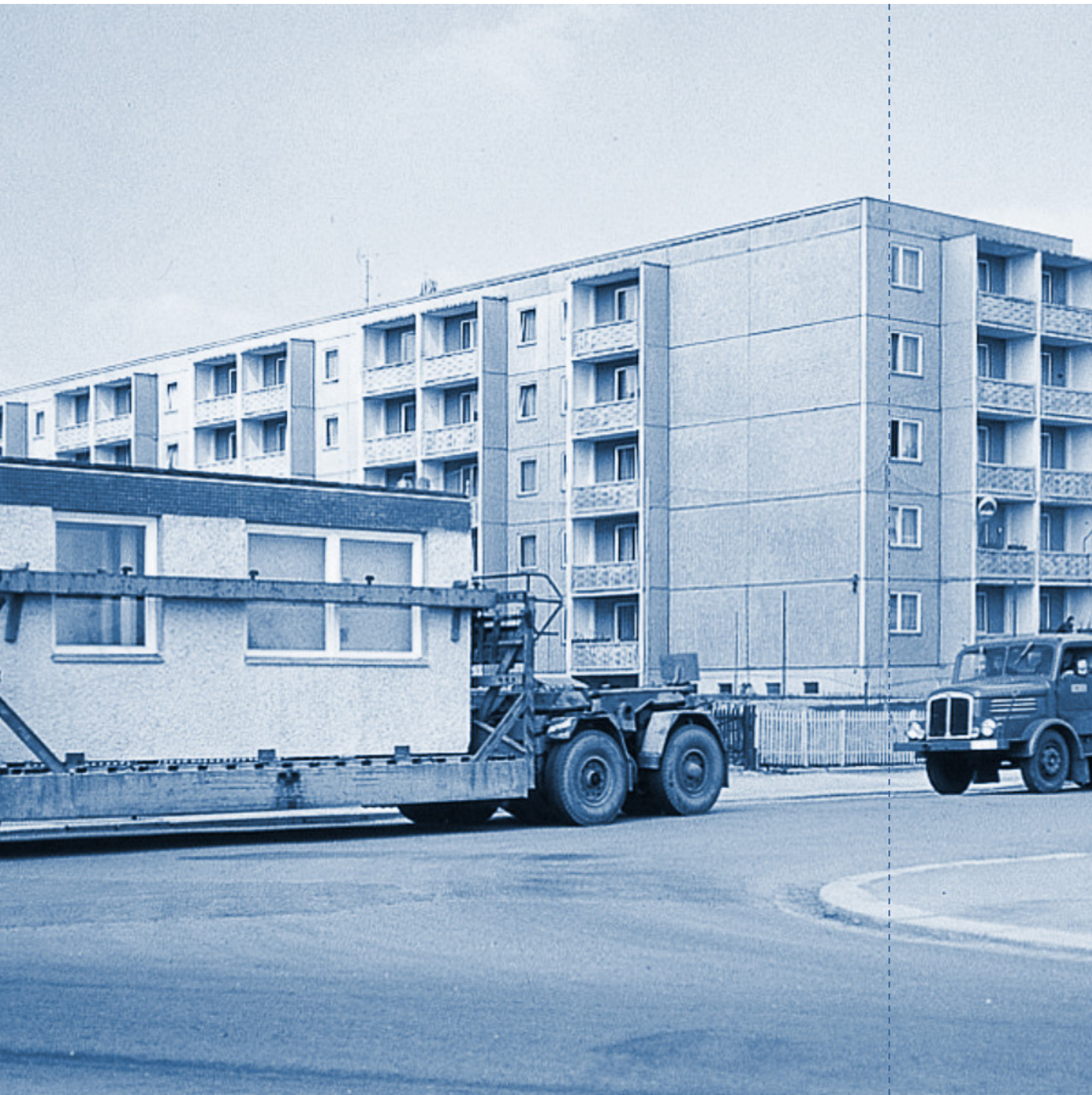
Panelka under construction
