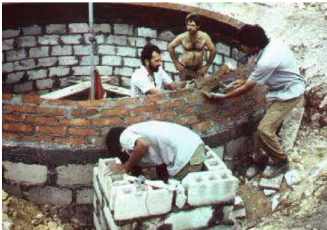
Figure 3.5: Masonry construction of a 30\text{ m}^3 dome. Retrieved from: [67]
