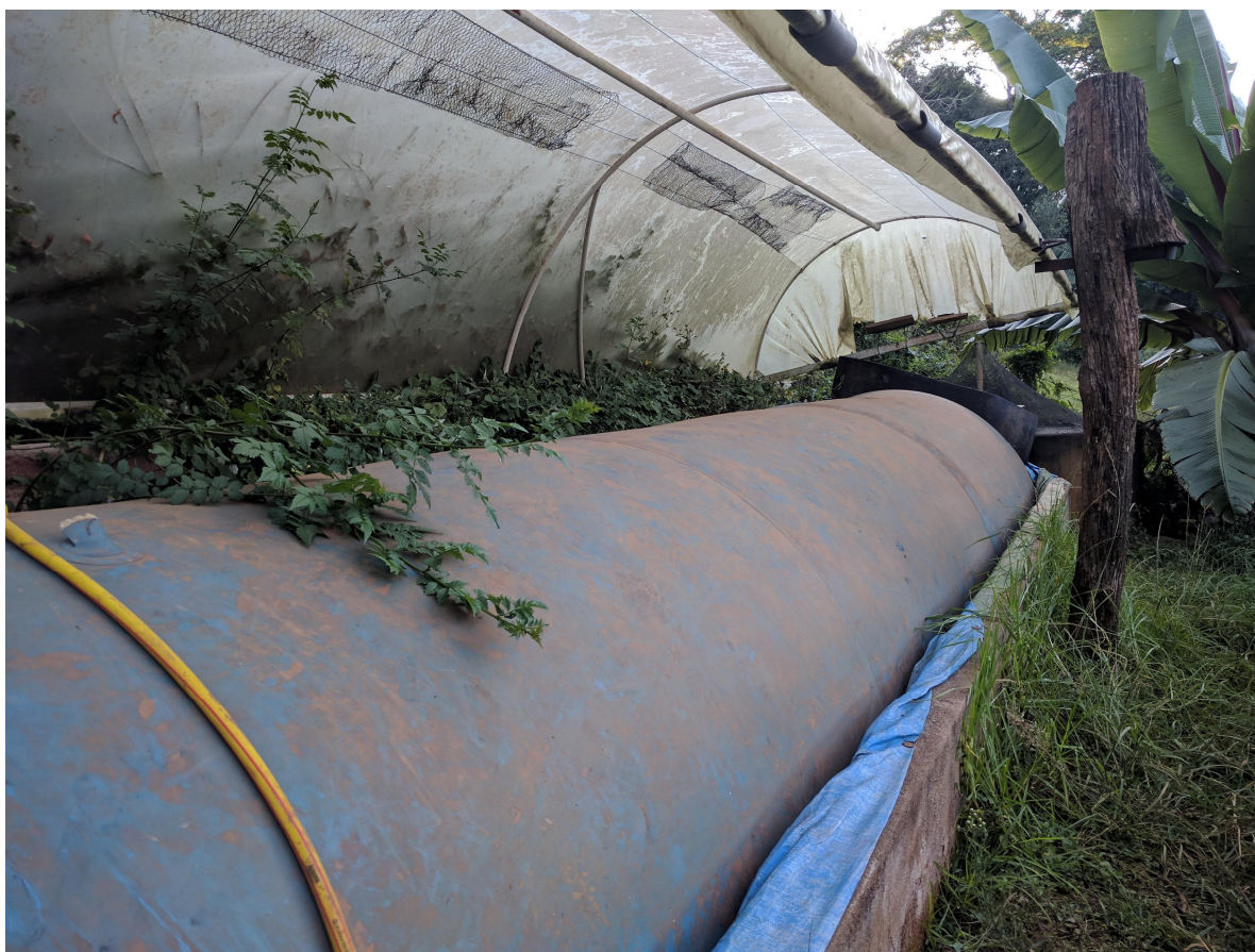
Figure 4.17: Plastic tubular dome digester in Limpopo.
