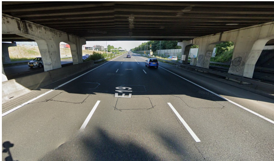
Figure 6.5: Picture of the loop detectors upstream of the on-ramp (Google, 2020b)
