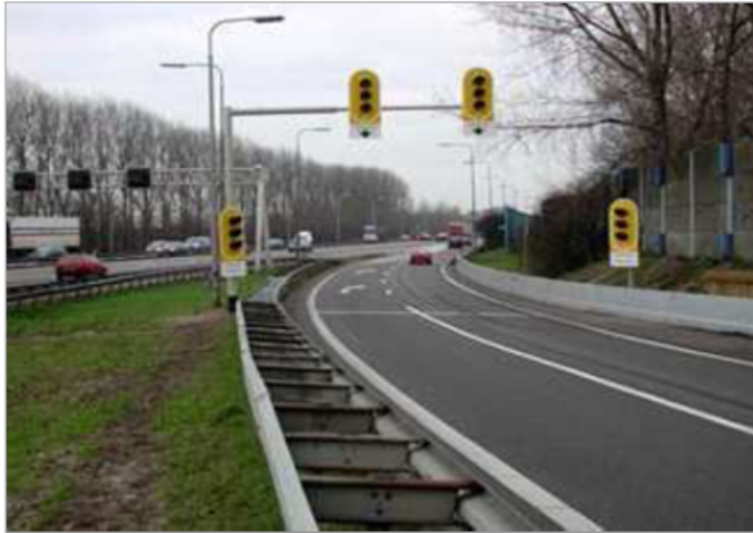
Figure 1.1: Ramp metering system in the Netherlands, A2 Maarsse-oost (Middelham and Taale, 2006)
