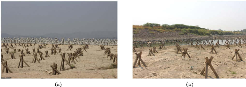
Figure 3.2: Scour and deposition patterns around partially-buried porcupines at two locations in Sagaing Channel (a) facing east (flow from right to left), and (b) facing west (flow from left to right)
