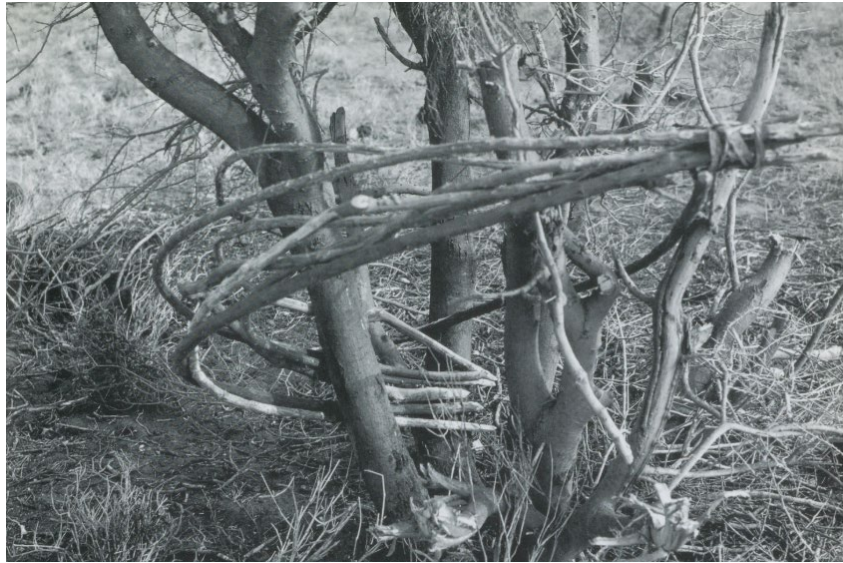
Figure 6 ~ Accacia roots tied around its trunk to create the dome shape for the Dhigo 45
