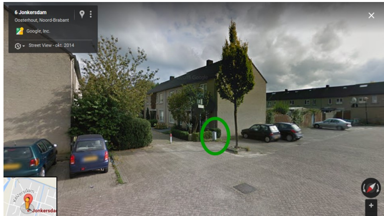
Figure 5-4: The house with the street cabinet next to it.
