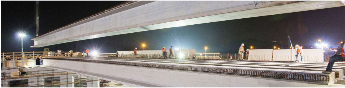
Figure 1, concrete bridge using girder beam, under construction (Haitsma Beton B.V., n.d.)
