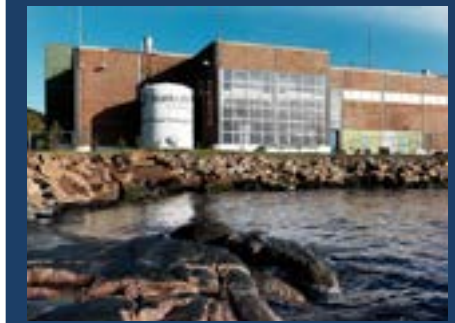
Figure 121. Image of the world's first osmotic energy plant in Tofte, Norway (Clark, 2013).
