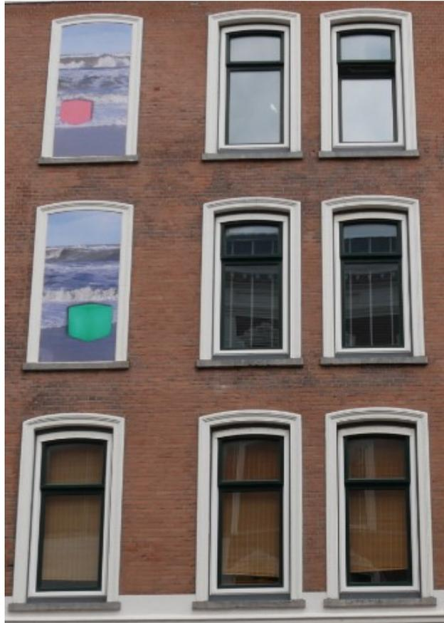
Figure 28: Facade 2 with fake window frames
