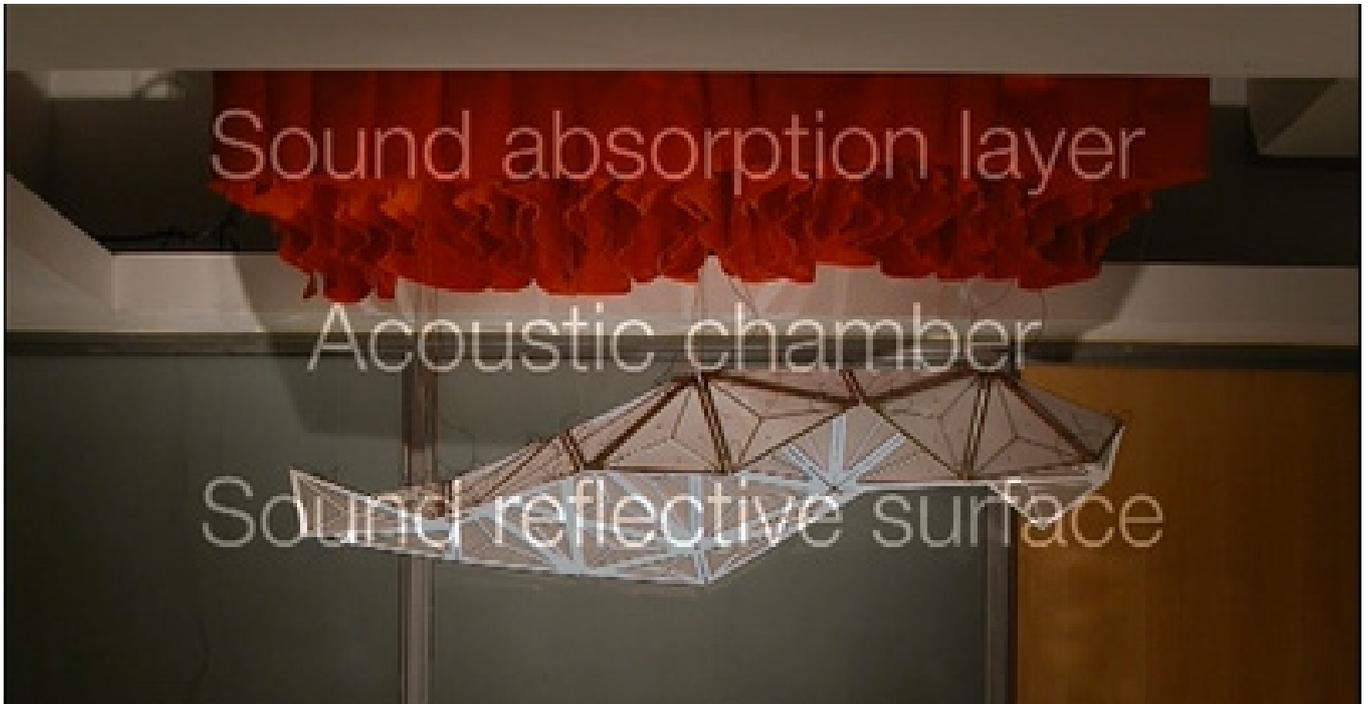
Figure 4.24 : Tuneable Sound Cloud (Fishtnk Design Factory)
