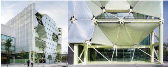
Figure 4.19 : ETFE cushion panels on ICT Medi Building (Poli, n.d.)
