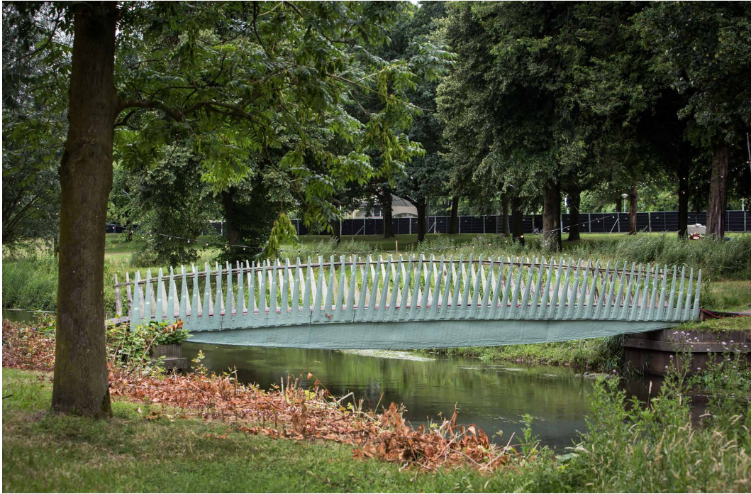
FIGURE 5.1 The bio-composite footbridge, 18 months after the installation across the river Dommel. R. Blok, J. Smits et al., Eindhoven University of Technology & Delft University of Technology, (2017). Photo by Heijmans (2018).
