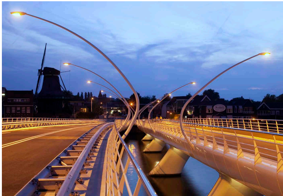
FIGURE 2.14 Light masts define the space and viewing directions. They emerge from the void in order not to obstruct the outward view. Royal HaskoningDHV, Joris Smits et al. (2013). Photo by Luuk Kramer 2009.
