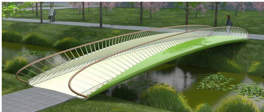
FIGURE 4.18 The Delft Design Composite Bridge. Royal HaskoningDHV & FiberCore, Joris Smits et al. (2008).
