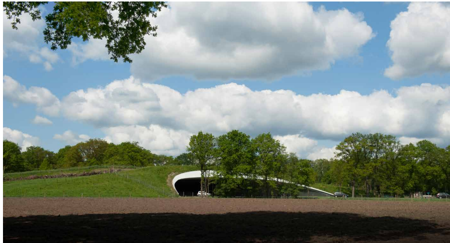
FIGURE 2.18 The wildlife crossing at Rijssen. Nature has the supremacy, in the form of soil and vegetation; the road is just a perforation of the earth, a guest that is temporally tolerated underneath it. Royal HaskoningDHV, Joris Smits et al. (2014). Photo by Jane van Raaphorst 2014.
