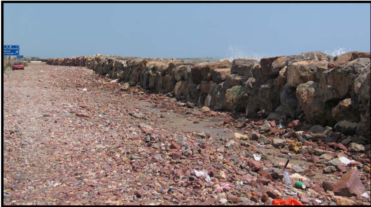
Figure A2.4. New motorway coastal defence.
