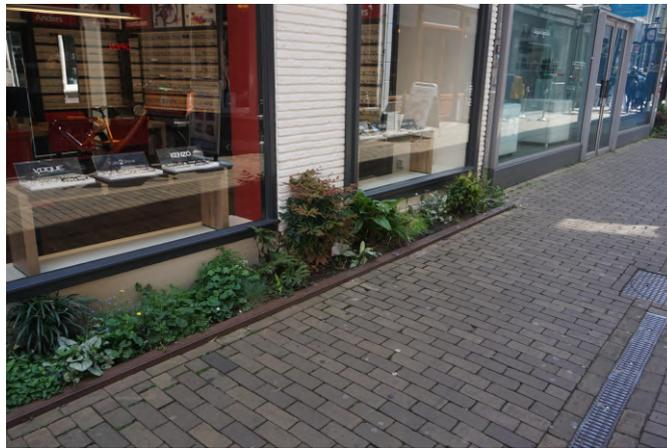
**Figure 5.10:** *Case #30: In this Case a façade garden is visible. Greenery traditionally have been separated from roads by raised sides (embedded practice). However, the raised sides in this Case make transport of water towards the facade garden impossible, whereby the facade garden can perform a minimal functionality.*
