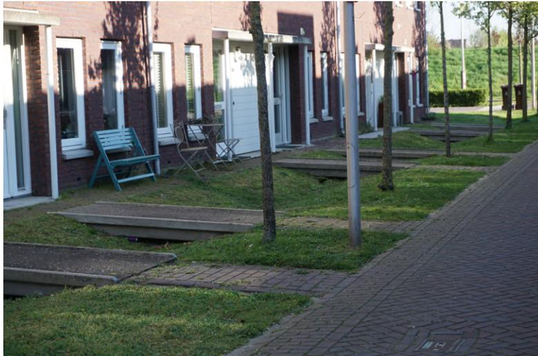
**Figure 5.15:** *Case #26: Vegetated swales are constructed in front of houses. However, these swales cannot be maintained properly, because mowing machines raise small stones that damage windows. Therefore, the maintenance becomes a time consuming and expensive matter.*
