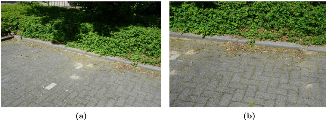
**Figure 5.20:** *Case #32: In this area porous pavement has been applied at streets and parking spots. When vegetation is constructed next to porous pavement, it happens that the porous pavement is blocked by leaves or dirt. This requires regular maintenance. However, operators are yet unfamiliar with the regular maintenance needs.*
