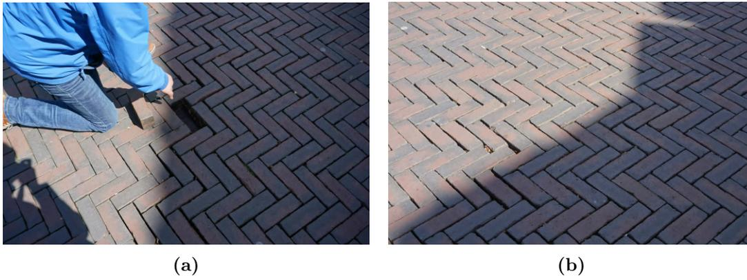
**Figure 5.12:** Case #29: The filling between the joints of permeable pavement bricks vanishes due to the load of cars and cleaning practices. There exists a lack of knowledge about the effects of other urban systems on the permeable pavement.
