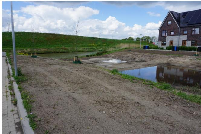
**Figure 5.18:** *In the sketch design phase it was decided to place the bioswale 30 cm higher, creating a playground for children that would be flooded two or three times a year at most. Due to a new staffing in the subsequent design phase that did not know the old principles, it was thought that the bioswales should be laid deeper so that there would always be water in the bioswale. The residents complained because they were promised a playground.*
