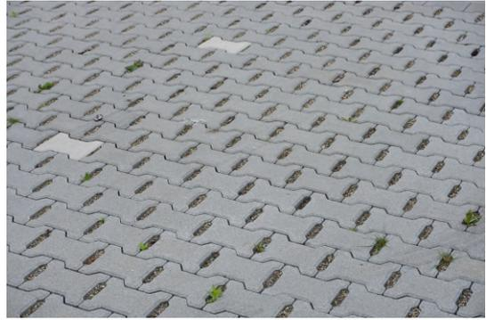
**Figure 2.11:** *Permeable pavement constructed at parking places in Zwolle*
