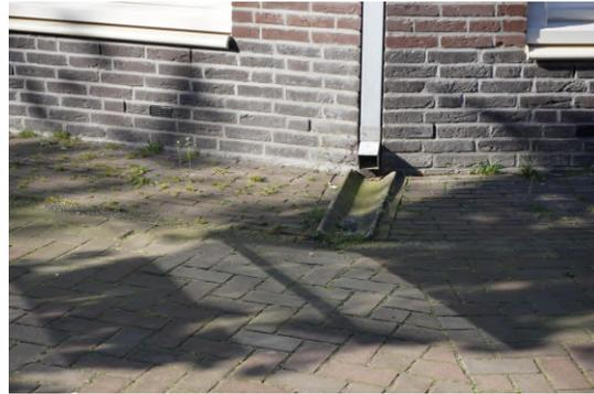
**Figure 2.5:** *Above-ground drainage from the house almost directly on the street*
