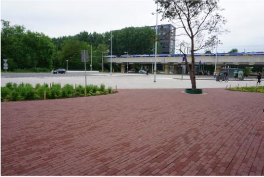
**Figure 2.10:** *Permeable pavement implemented on a square in Amsterdam*
