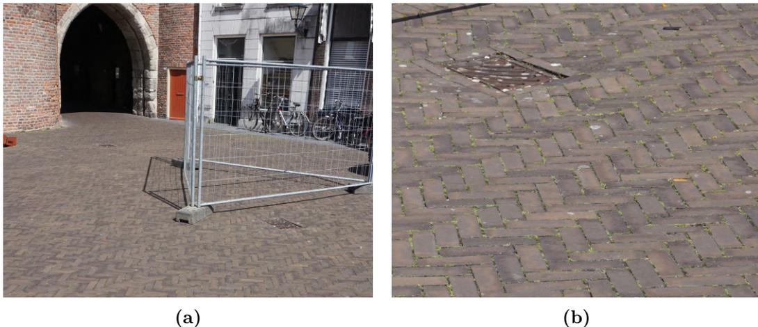
**Figure 5.16:** *Case #28: Next to the permeable pavement, a gully was constructed in order guarantee the drainage of stormwater. In order for the stormwater to reach the gully, the surface was laid with a small gradient towards the gully. Therefore, the water partly infiltrates via the permeable pavement and partly is drained via the stormwater sewer system.*
