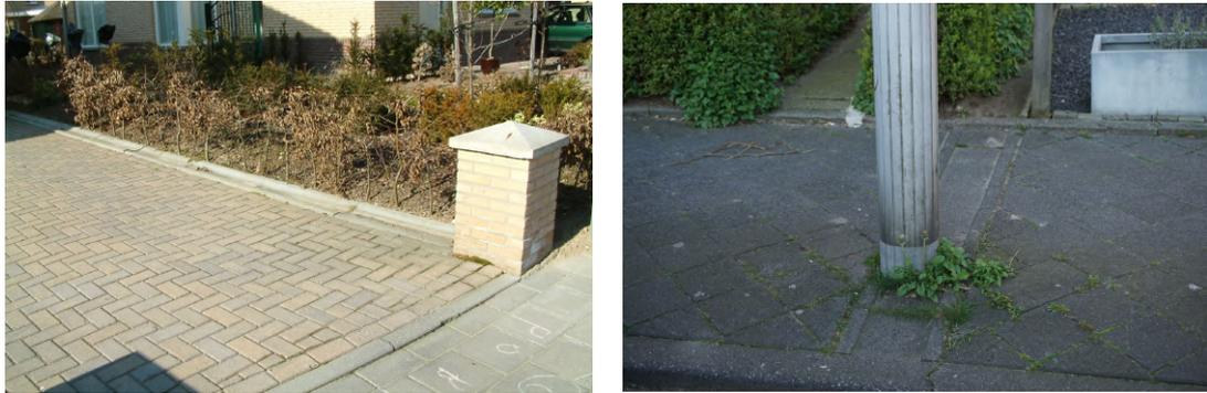
(a) Case #13: Structure blocking open gutter (b) Case #7: Lamppost blocking open gutter
