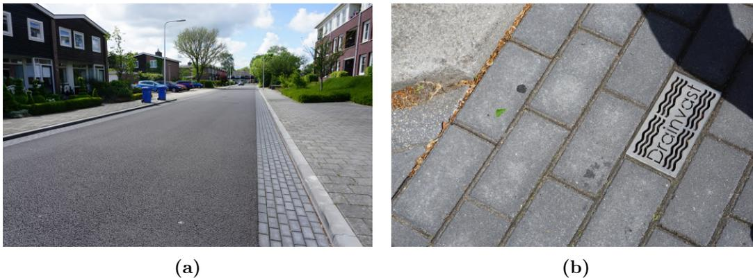
**Figure 5.13:** Case #33: The permeable pavement with drainvast joints aims to infiltrate the stormwater falling on the street. After small rainfall events, water remains present for at least one hour. There existed an incomplete knowledge about the internal technical processes. It is expected that the slow infiltration can be caused by the connection between the split and the granulate layer.
