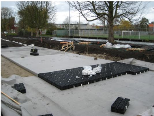
**Figure 2.6:** *Construction of infiltration crates at the Emmastraat in Gouda*
