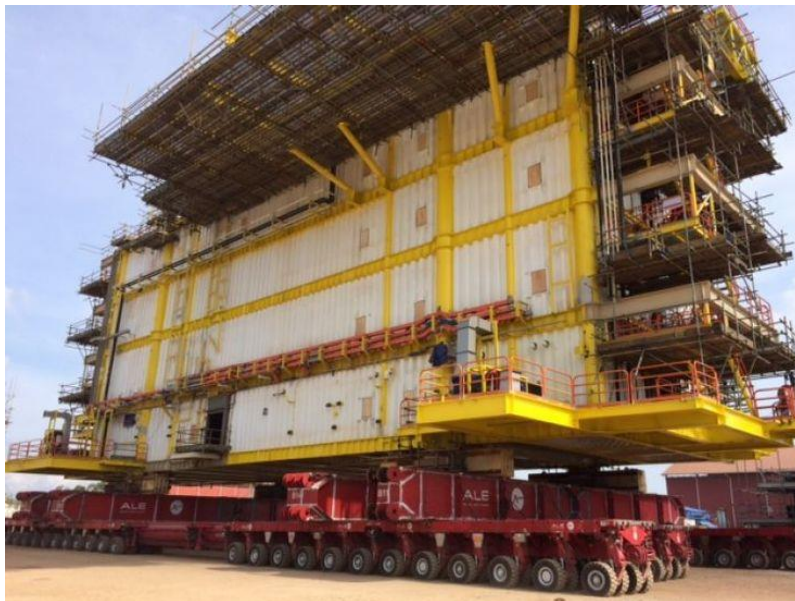
Figure 2-2 Trailered load-out
