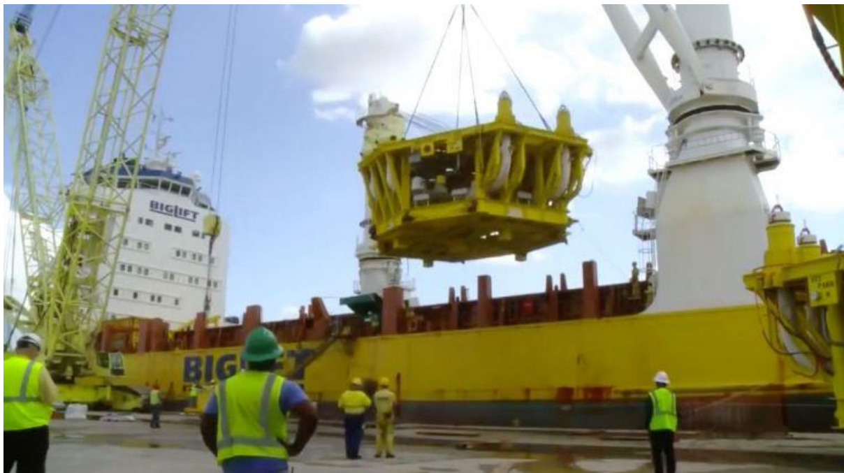
Figure 2-1 Lifted load-out
