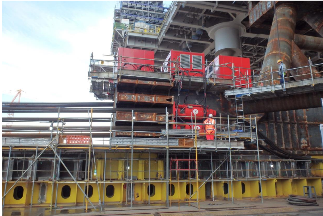
Figure 2-4 Strand jack attachment front skidbox
