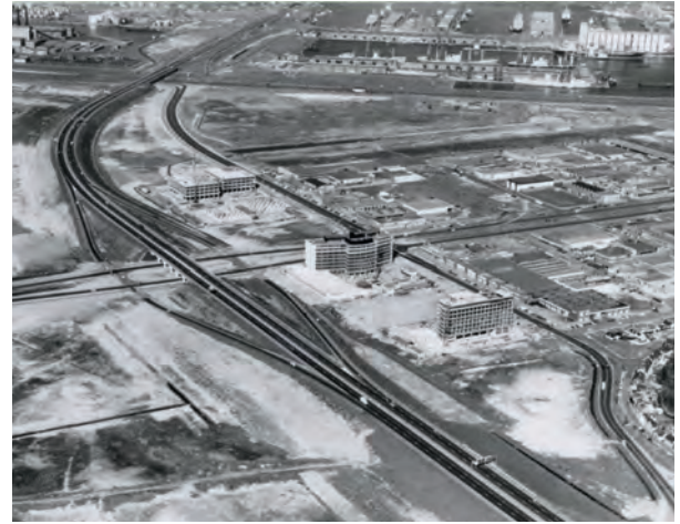
Figure 2.8. Construction of Bos en Lommerplein, 1968 (Ring West). This is the only part where buildings are used as sound barriers
