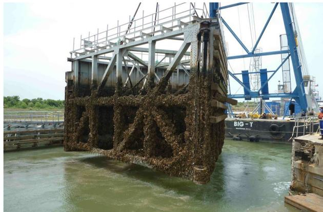
**Figure 5.3:** Oyster growth on sector gates at Brazos River Floodgates Project, Freeport, TX (USACE, 2011).
