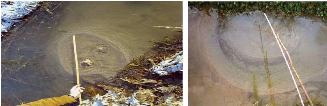
Figure 1-1 two sand boils as result of the piping process (Wejers, 2010)
