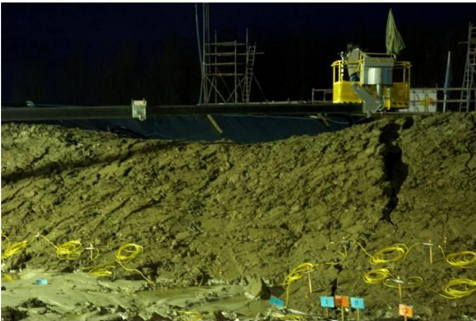
Figure E-6 failure of de IJkdijk because of piping (de Bruijn, 2009)
