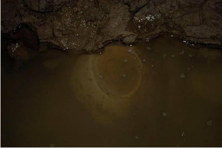
Figure E-5 a sand boil at de IJkdijk (de Bruijn, 2009)
