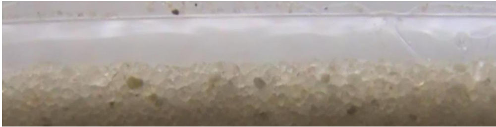
Figure 3-19 the bottom of the channel after the channel is completely cleared Q17 04:04
