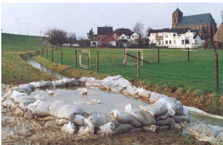
Figure 1-7 sand bags around a sand boil (" opkisten ") (Weijers, 2010)
