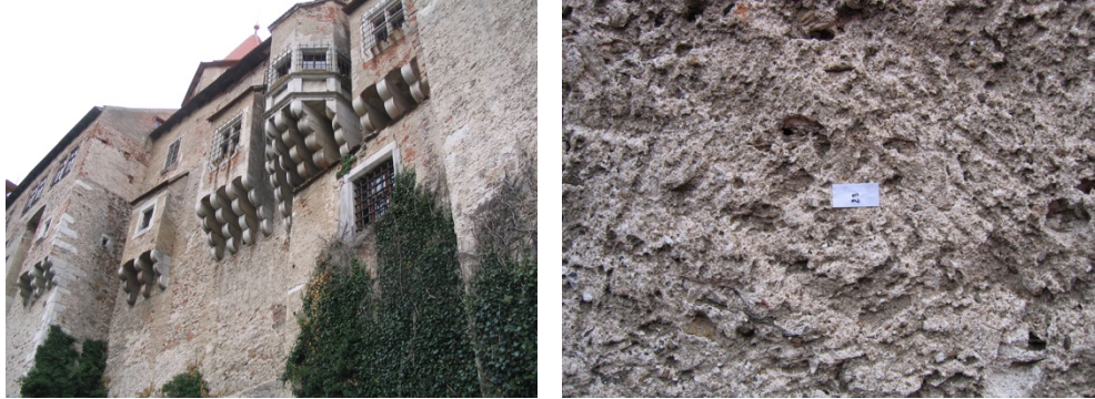
Fig. 3.1 Disintegrated and partly detached render on Renaissance castle masonry (l). Peeling tests performed before the consolidation treatment (r), Pernštejn castle (Czech Republic)
