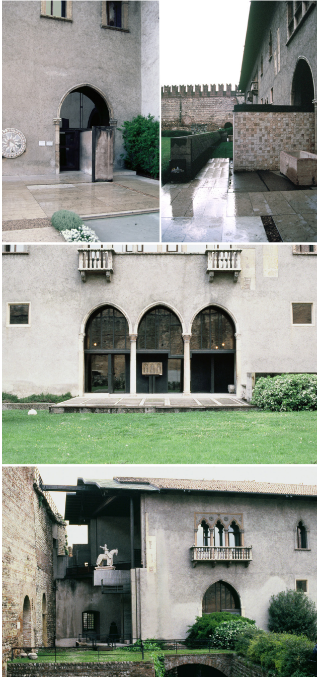
Fig. 9: Carlo Scarpa, intervention in Castelvecchio, Verona (1958–64). From top to bottom and from left to right: entrance crossed by an L-shaped wall and spolium to the left; view along the façade with projecting volume, low wall, and spolium in the foreground; central loggia with asymmetrical, recessed glazing, spolium and terrace; western extremity of the north volume, with Cangrande, communal wall to the left and Roman moat in the foreground. Photos: author.
