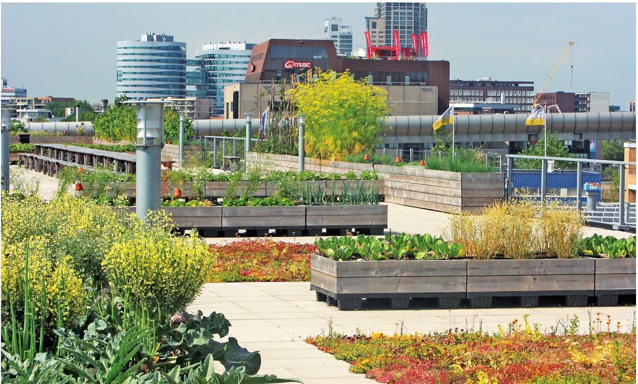
Roof top (zinco-greenroof.com)
