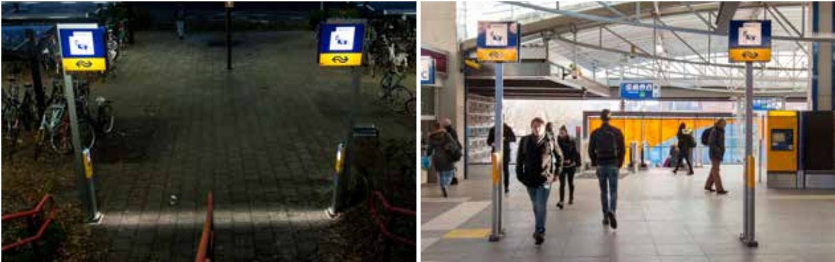
Figure 45: Veenendaal-De Klomp and Den Bosch stations with the test installation.
