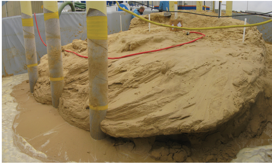
Figure 2 The cemented sand body in the first field scale experiment on BioGrout: a ground improvement method based on microbial induced carbonate precipitation by urea hydrolysis.
