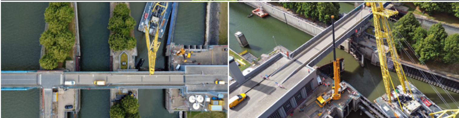
Prinses Marijkesluis, Rijswijk (Gelderland): the renovation project involves major upgrades to the lock gates, bridge structures and control systems, as well as concrete repairs, so the lock can continue to operate safely for the next 30 years. A floating crane lifts the 40-ton lock gate during the renovation. [© Rijkswaterstaat] / Oosterscheldekering in Zeeland: preservation of the gates of the storm surge barrier with an engineering & construct contract. [© Rijkswaterstaat, Paul van Baardwijk]
