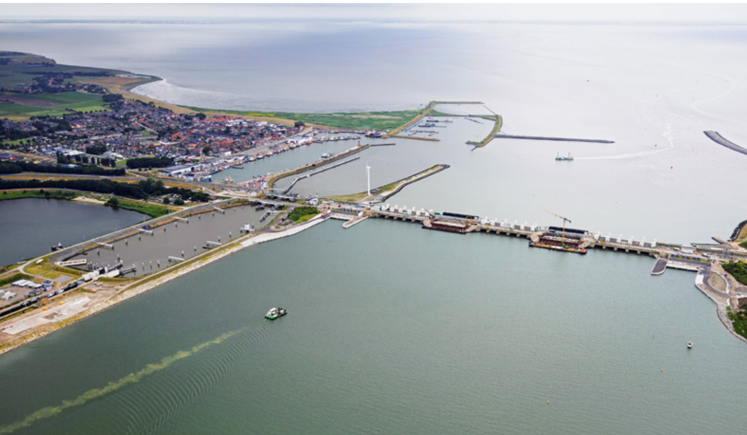
Reinforcement and renewal of the Afsluitdijk: Kornwerderzand sluice complex with sea lock, Lorentz sluice gates and the new Fish Migration River (under construction) as seen from the Wadden Sea. / Den Oever sluice complex with sea lock, two new pump stations, and additional sluice gates (under construction) next to the existing Stevin sluice gates, as seen from the IJsselmeer. [© Levvel, Topview Luchtfotografie]
