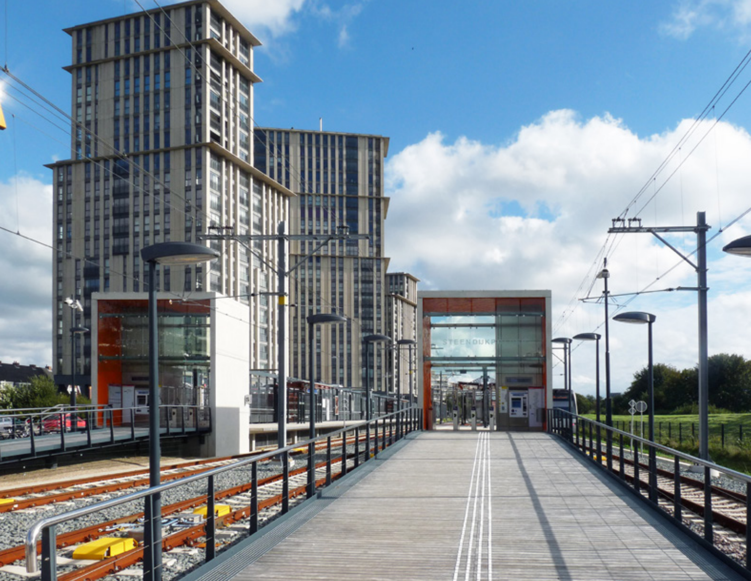
Figure 5. Actual realisation of metro station Steendijkpolder in Maassluis as a new stop with new apartment buildings as an example of urban development. [CC Smiley toerist]
