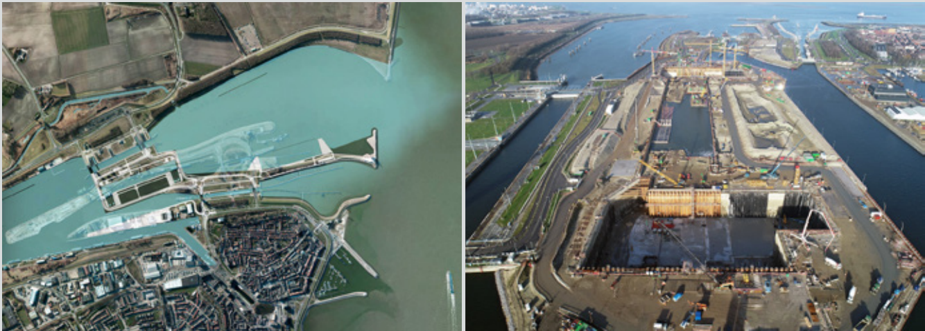
Aerial view of the Terneuzen lock complex with the old situation indicated in the background. / The 25-metre deep building pit for the inner lock head and the lock chamber of the Nieuwe Sluis. [© project Nieuwe Sluis Terneuzen]
