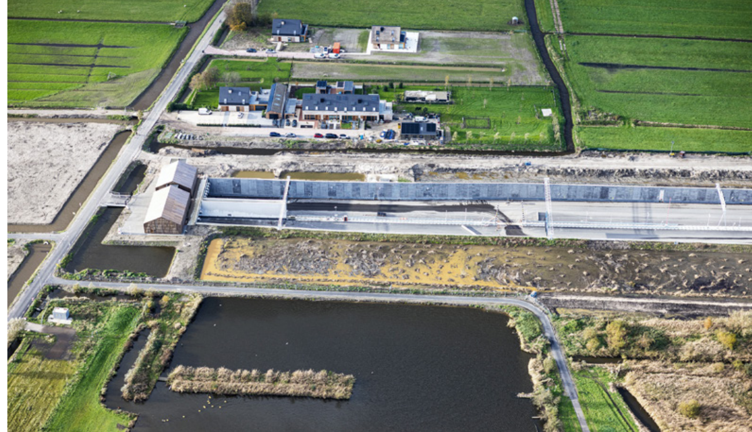
Figure 10. Construction of the Holland tunnel near Zuidbuurt. [© Rijkswaterstaat, Topview Luchtfotografie]
