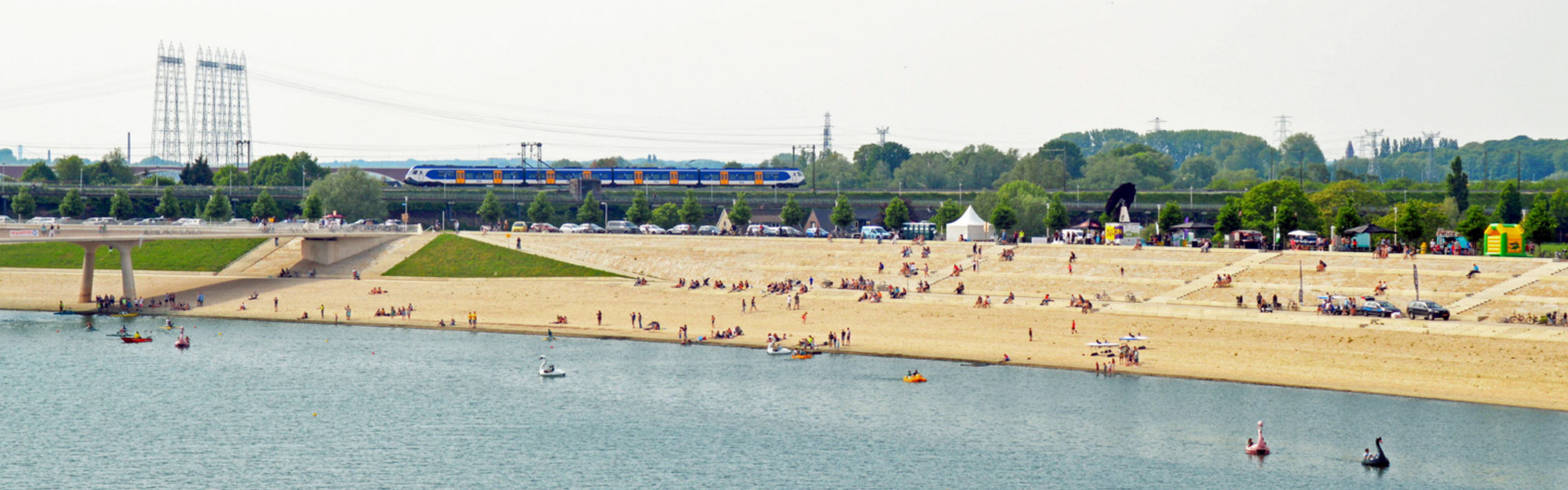
Figure 4. Nijmegen, Lent, Gelderland: dike movement and a new canal, Spiegelwaal, for lowering the water level of the nearby Waal River, and a sloping and, wide bank for recreation. [CC Roger Veringmeier]
