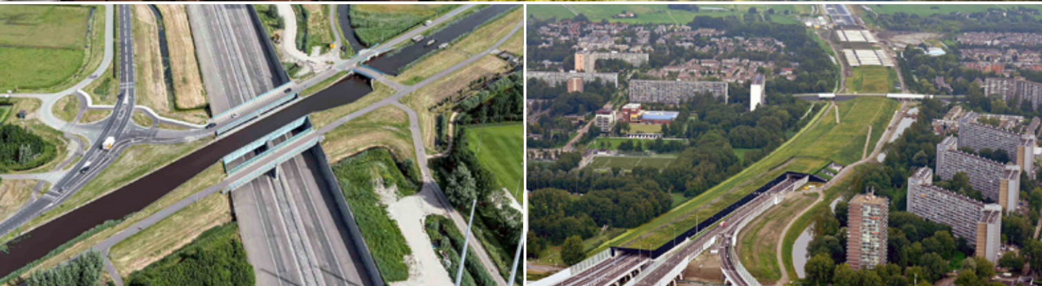
A4 Delft-Schiedam, South Holland: sunken motorway through the Midden-Delfland polder area, minimizing noise and visual disruption and maintaining waterways, with the Kethel land tunnel at Schiedam. [© Jeroen Musch (top) / © Rijkswaterstaat, Joop van Houdt (middle)] / Below: lowered lightning to reduce spill-over in the landscape. [© Heijmans, Marc Blommaert]
