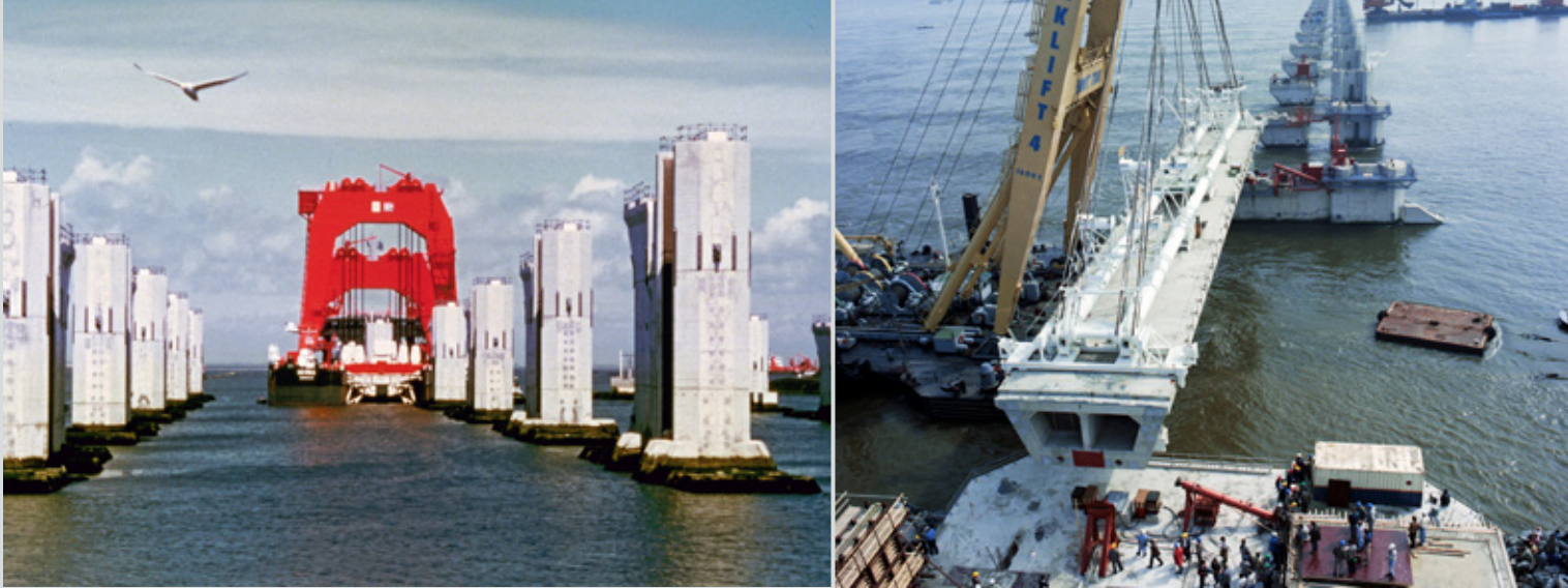
The Ostrea, a dedicated vessel for lifting and positioning piers to their location. / Placement of a traffic shaft for road support, housing the drive and control equipment for the gates. [© Rijkswaterstaat, Harry van Reeken] / Below: piers and gates and traffic shaft with the road on top. [© Rijkswaterstaat, Joop van Houdt] / Roompot ship lock for recreational boats with the N57 motorway at the artificial island of Neeltje Jans. [© Rijkswaterstaat, Joop van Houdt] / Aerial view of the Oosterscheldekering as seen from Noord-Beveland with the Roompot barrier, Neeltje Jans, the Roompot ship lock and the former working ports Mattenhaven and Betonhaven. [© Siebe Swart]
