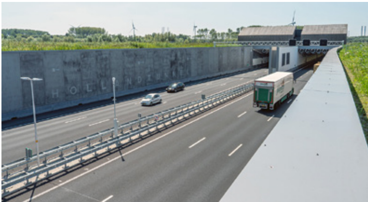
Figure 6. The immersion of one of the concrete tunnel elements of the Maasdelta tunnel. [© Rijkswaterstaat, Topview Luchtfotografie] / Figure 7. Tunnel construction work on both the north and south banks. [© Rijkswaterstaat, Topview Luchtfotografie] / Figure 8. The sunken road along Krabbeplas and entrance to the Holland tunnel with the ventilation systems 'disguised' as sheds in the Zuidbuurt. [© Stan Wanders] / Figure 9. Entrance to the Maasdelta tunnel towards the A15 on the south bank. [© Stan Wanders]
