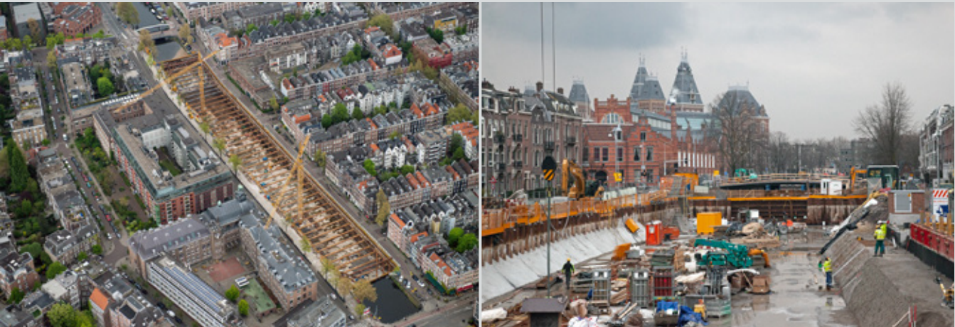
Construction pit. [© Max Bögl] / Building equipment on the roof and construction of the car entrance at Ruysdaelkade. [© ZJA Architects & Engineers]
