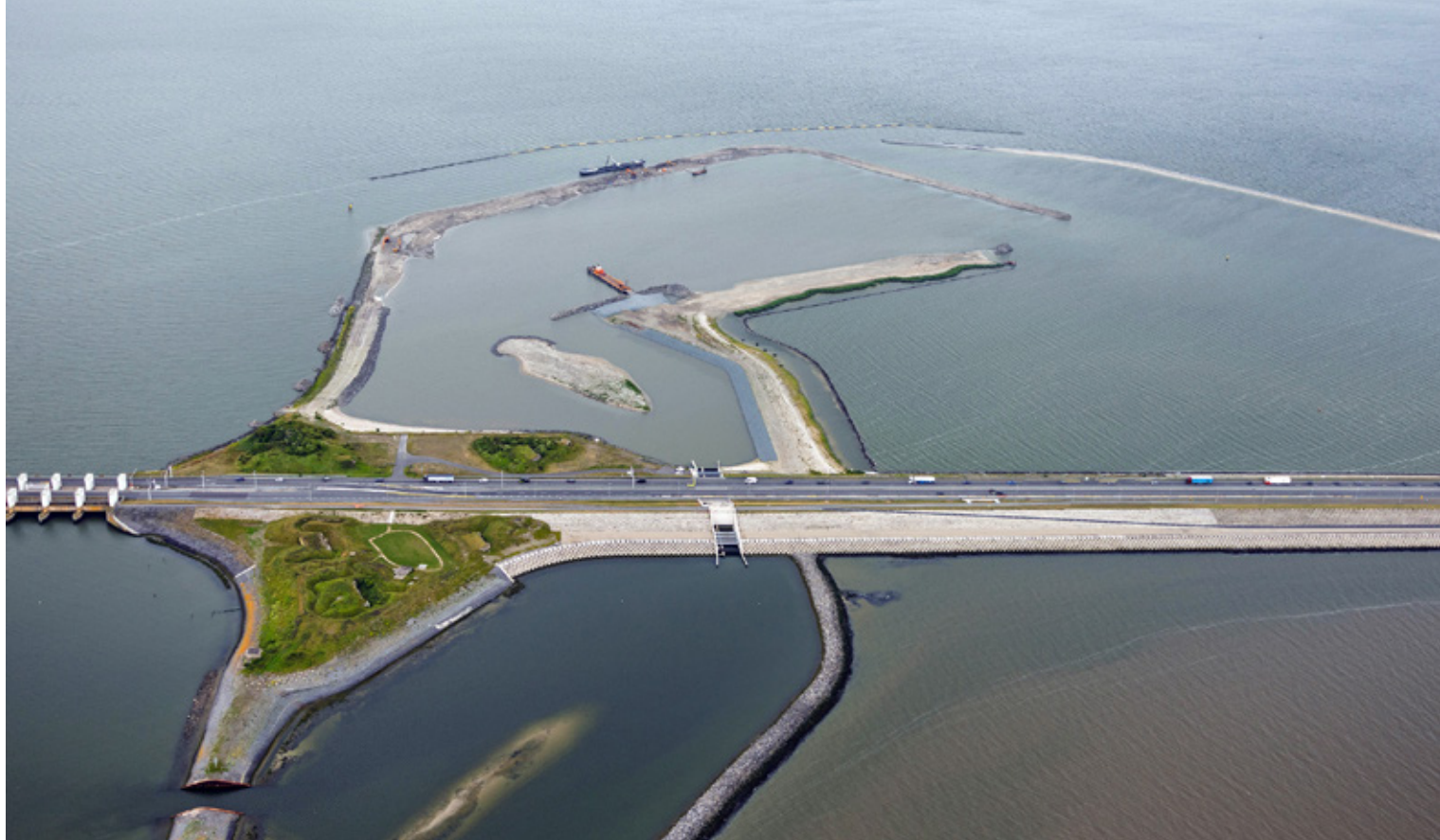
Figure 8. Casemates and culvert for the fish passage through the Afsluitdijk with the Fish Migration River under construction. [© Levvel, Topview Luchtfotografie]
