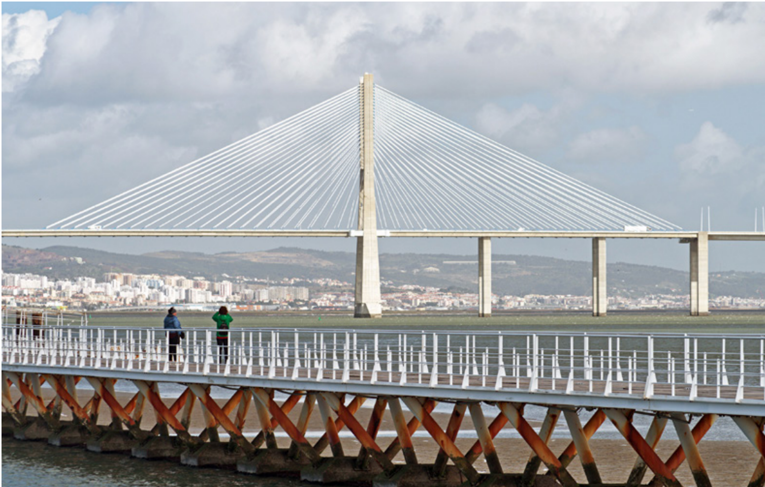
Figure 3. Most common bridge typologies. [© Ney & Partners] / Lissabon: cable-stayed section of the Vasco da Gama bridge designed by Armando Rito. The total length is 17,185 m of which 12,345 m for the bridge structure. The width is 30 m and its navigation clearance is 47 m for the main bridge. The longest span is 420 m. [CC Rob Oo]
