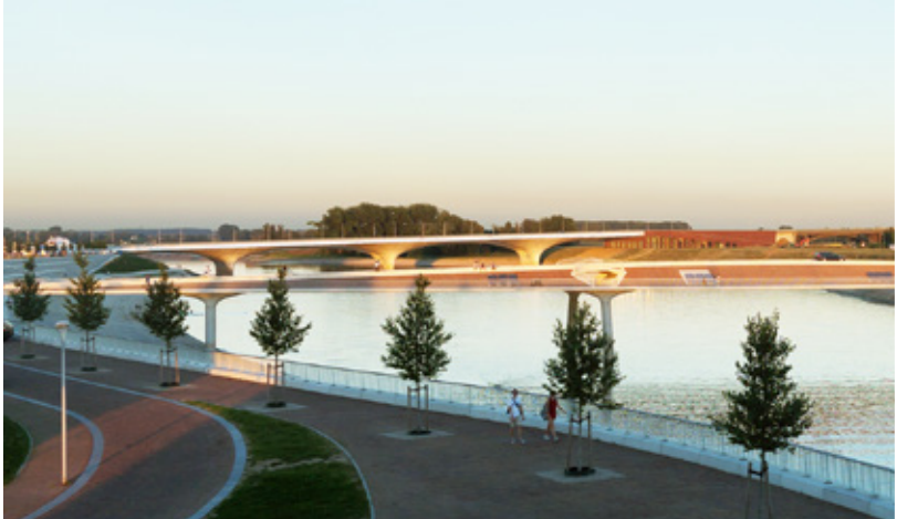
The Lentloper, Nijmegen is home to the largest colony of barn swallows in the Netherlands. The rebate between the underside of the bridge deck and the pillar was initially intended to compensate for intolerances of the slightly curved concrete deck in relation to the various pillars. Now it is an ideal place for nesting. Design by Ney & Partners. [CC Michiel Verbeek / © Ney & Partners]
