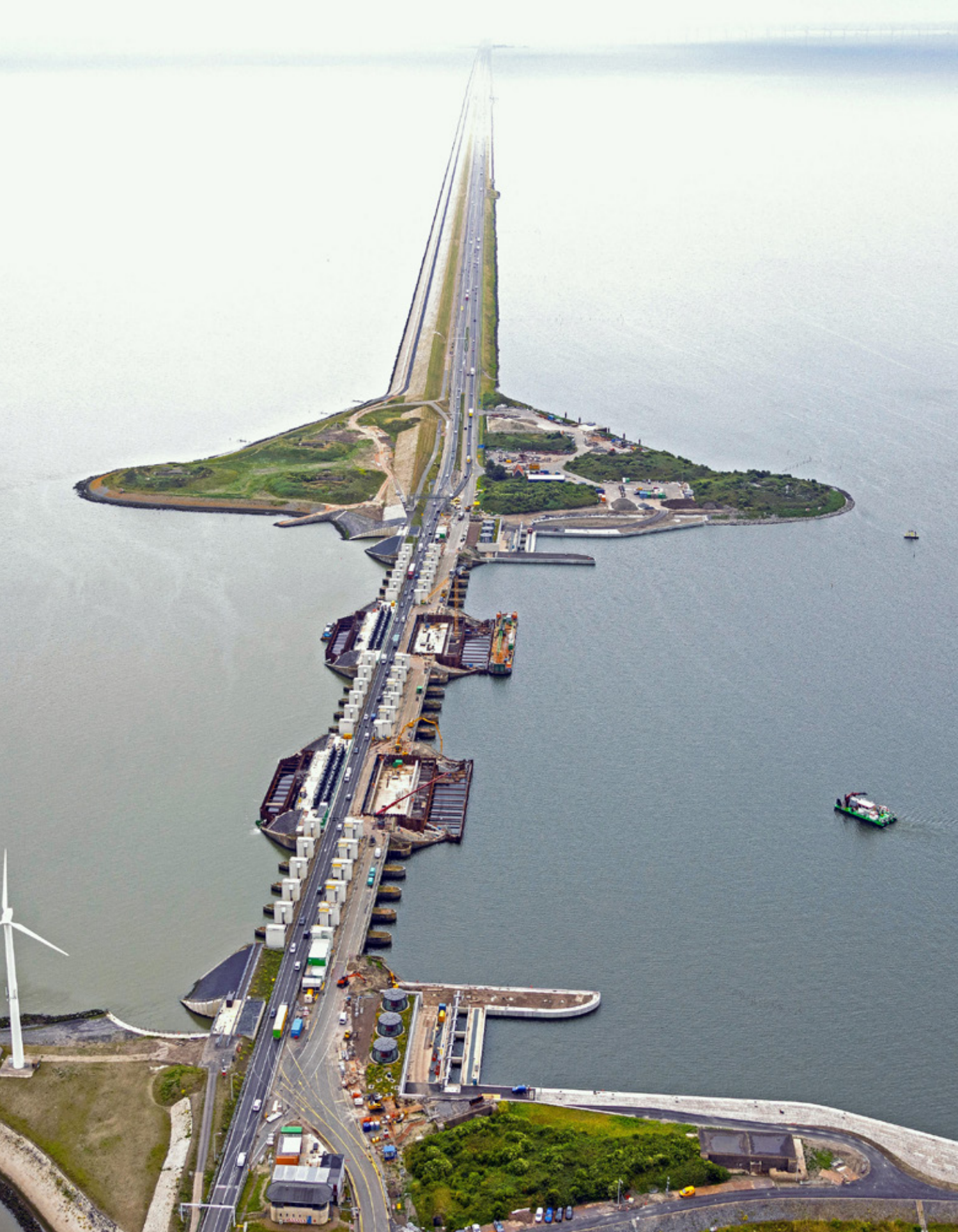
Figure 9. Aerial view on the Den Oever sluice complex and the Afsluitdijk in the direction of Friesland. [© Levvel, Topview Luchtfotografie]
