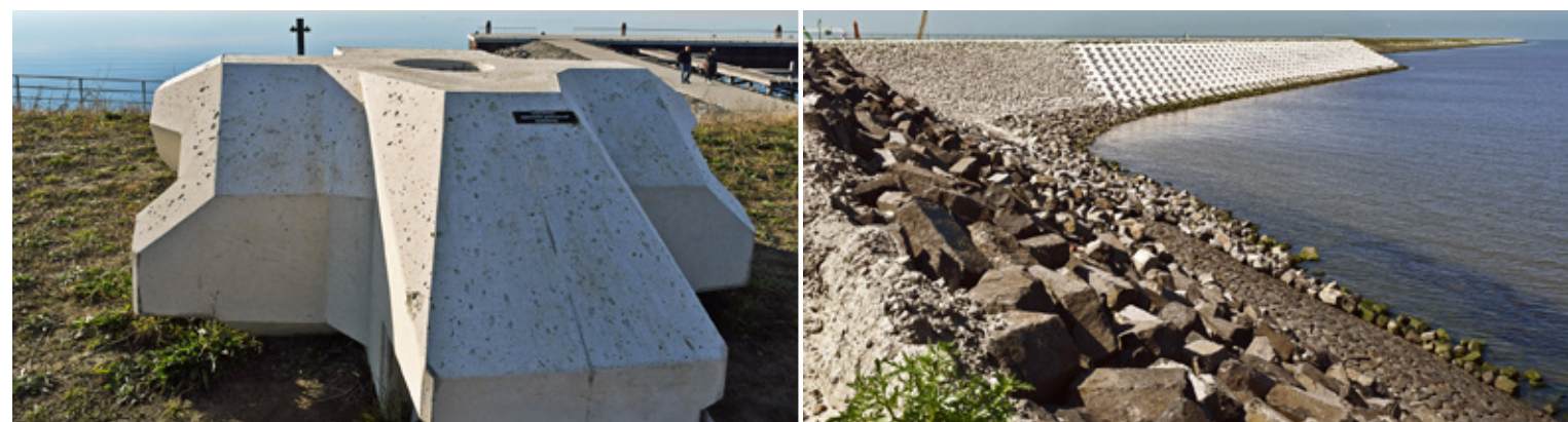
Figure 6. Left: newly developed Levvel bloc for reinforcement of the dike at the Wadden Sea side. [© Jan Wessels] / Right: application of Levvel blocs for the Fish Migration River. [© Rijkswaterstaat, Jan Wessels] / Figure 7. New pumps (left) at Den Oever sluice complex next to the existing sluice gates (middle). Additional sluice gates are under construction (right). This configuration is doubled within the entire complex. [© Levvel]
