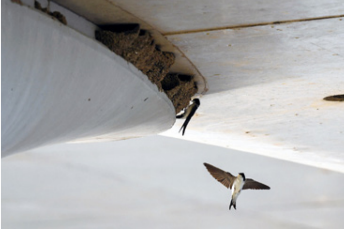
The Lentloper, Nijmegen is home to the largest colony of barn swallows in the Netherlands. The rebate between the underside of the bridge deck and the pillar was initially intended to compensate for intolerances of the slightly curved concrete deck in relation to the various pillars. Now it is an ideal place for nesting. Design by Ney & Partners. [CC Michiel Verbeek / © Ney & Partners]
