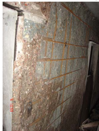
Fig. 1.5 Damage to the concrete structure of a car park in Rotterdam, the Netherlands after a fire on October, 1 st 2007 showing severe damage to the roof and spalling of the wall (pictures by Efectis).
