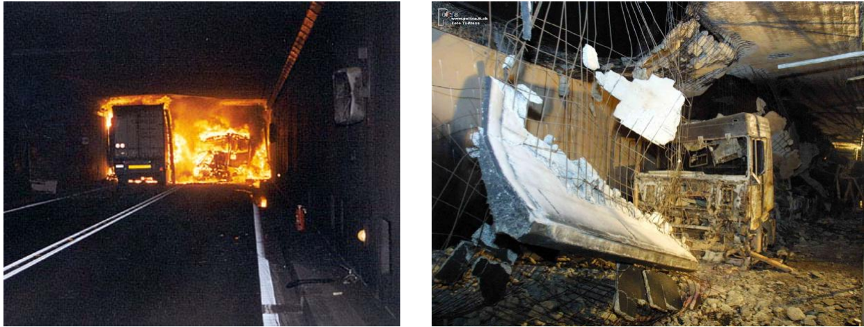
Fig. 1.4 Fire in the Gotthard tunnel between Italy and Switzerland on October, 24 th 2001 with partial collapse of the concrete roof (pictures by EPA (left) and by Ti-Press (right)).
