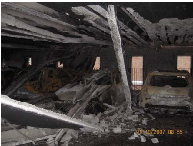
Fig. 1.5 Damage to the concrete structure of a car park in Rotterdam, the Netherlands after a fire on October, 1 st 2007 showing severe damage to the roof and spalling of the wall (pictures by Efectis).
