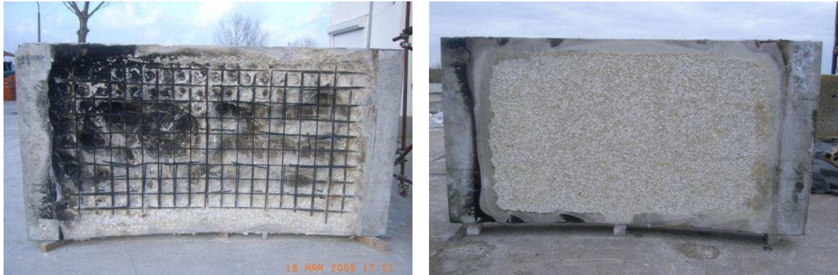
Fig. 2.29 Spalling damage to similar segments, without (left) and with (right) 2.0 \text{ kg/m}^3 of PP-fibres added to the C30/37 mixture. Both members were loaded to service life conditions during testing according to the ZTV-ING curve (Dehn, et al., 2010).
