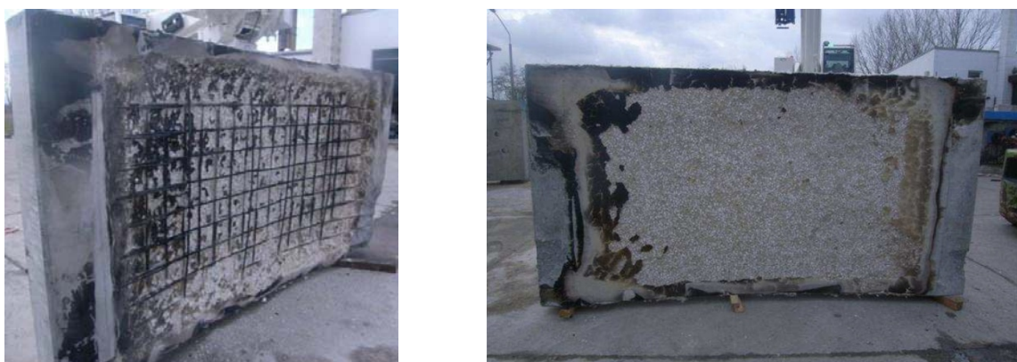
Fig. 2.28 Observed spalling damage to C30/37 tunnel lining segments made with limestone aggregate, without (left) and with (right) addition of 2.0 \text{ kg/m}^3 of PP-fibres. Both members were exposed to a ZTV-ING type of fire (Dehn, et al., 2010).
