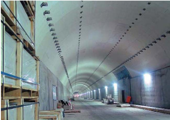
Fig. 1.13 Fire protection boards in the Elb tunnel in Hamburg, Germany (Promat International N.V., 2003).
