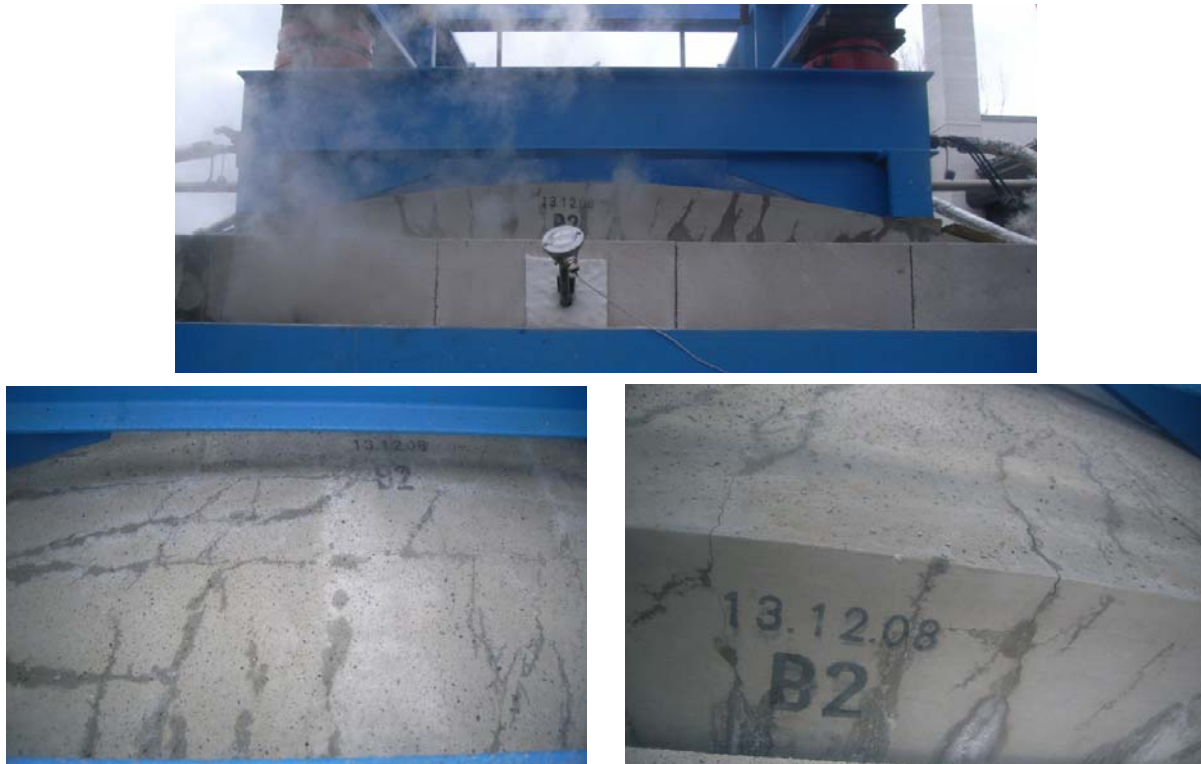
Fig. 2.19 Crack development observed during full scale fire testing of a tunnel lining segment with applied external loading (pictures by MFPA 7 ).
