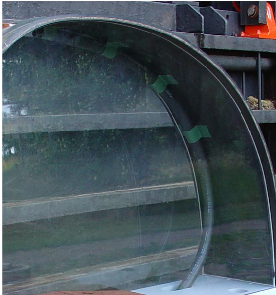
Figure 98: A part of an inflatable dam with an internal tube for pumping air out.
