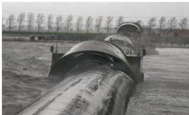
Figure 70: Shifting of the inflatable dam.
