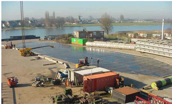
Figure 32: Unrolled sheet near the final location Ramspol (Photo: Bouwdienst Rijkwaterstaat).
