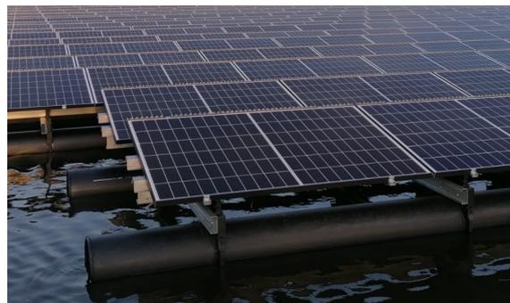
**Figure 2.5:** Floating Solar sealed plastic tubes [21]
