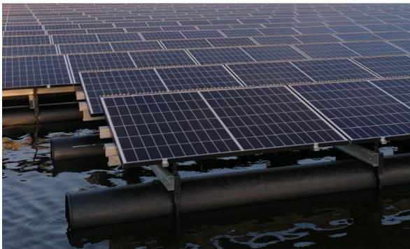
Figure 4.3: Floating Solar design [21]
