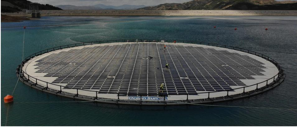
**Figure 4.8:** Ocean Sun, flexible membrane
